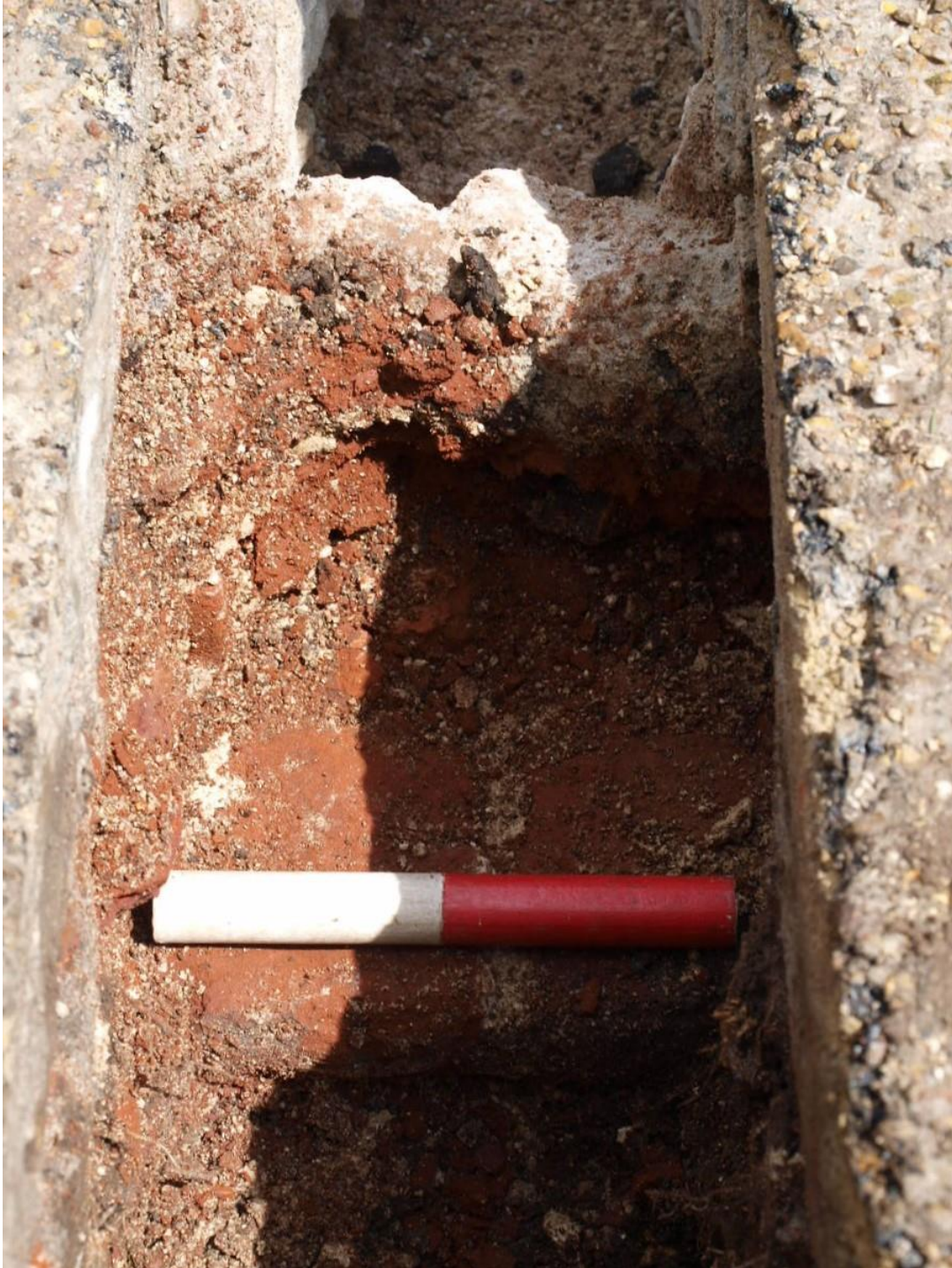
Plate 6. Wall [9] post-removal of two brick courses (0.20m scale)
