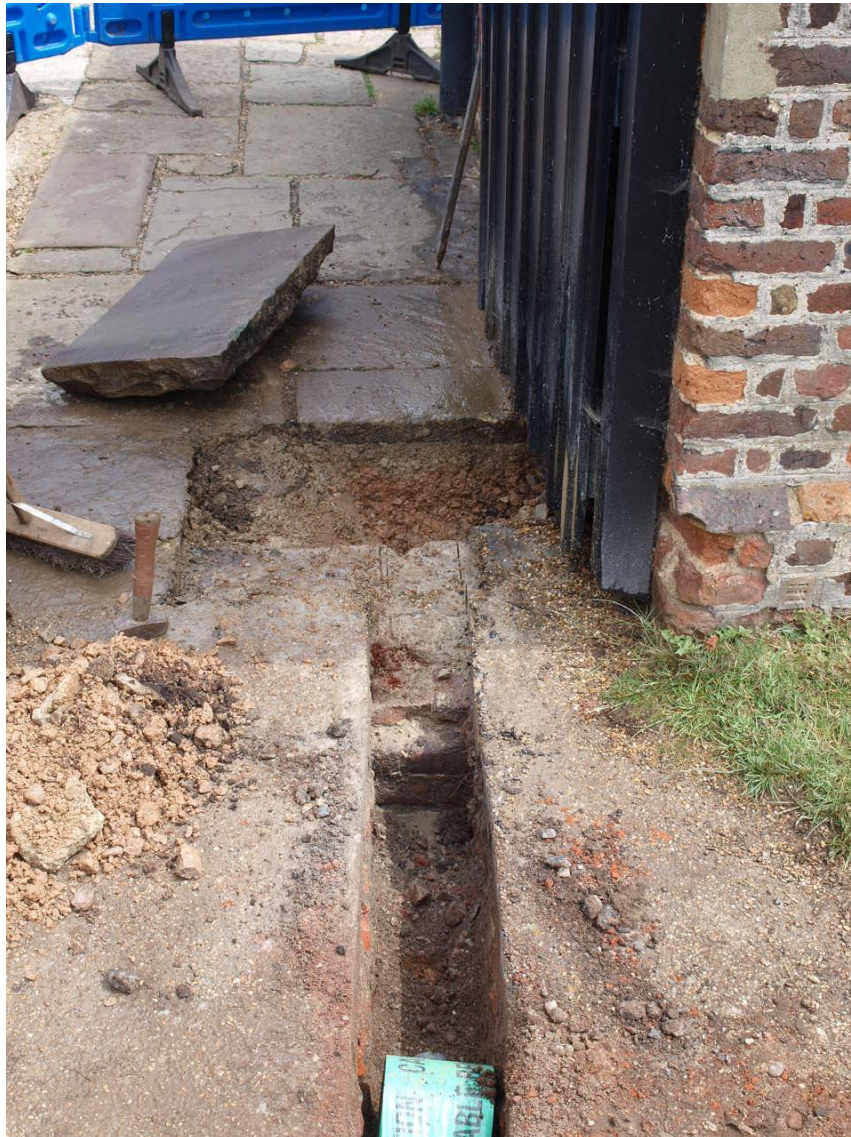
Plate 4. East facing photo showing wall [9] within the current doorway leading to the public toilets
