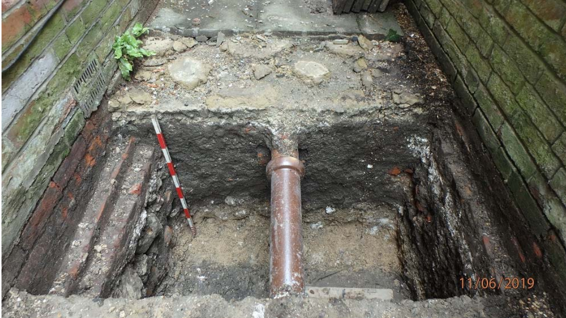
Plate 2 - South-east facing section of foundation trench 1, showing wall 003. Scale 1.0m.
