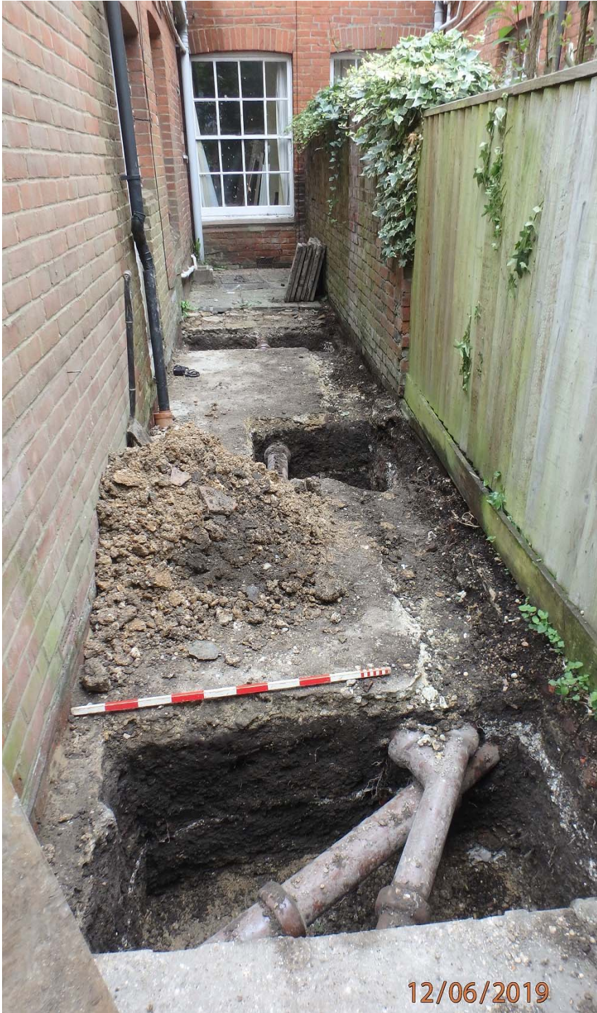
Plate 1 - Location shot of foundation trenches, view to north-west. Scale 1.0m.
