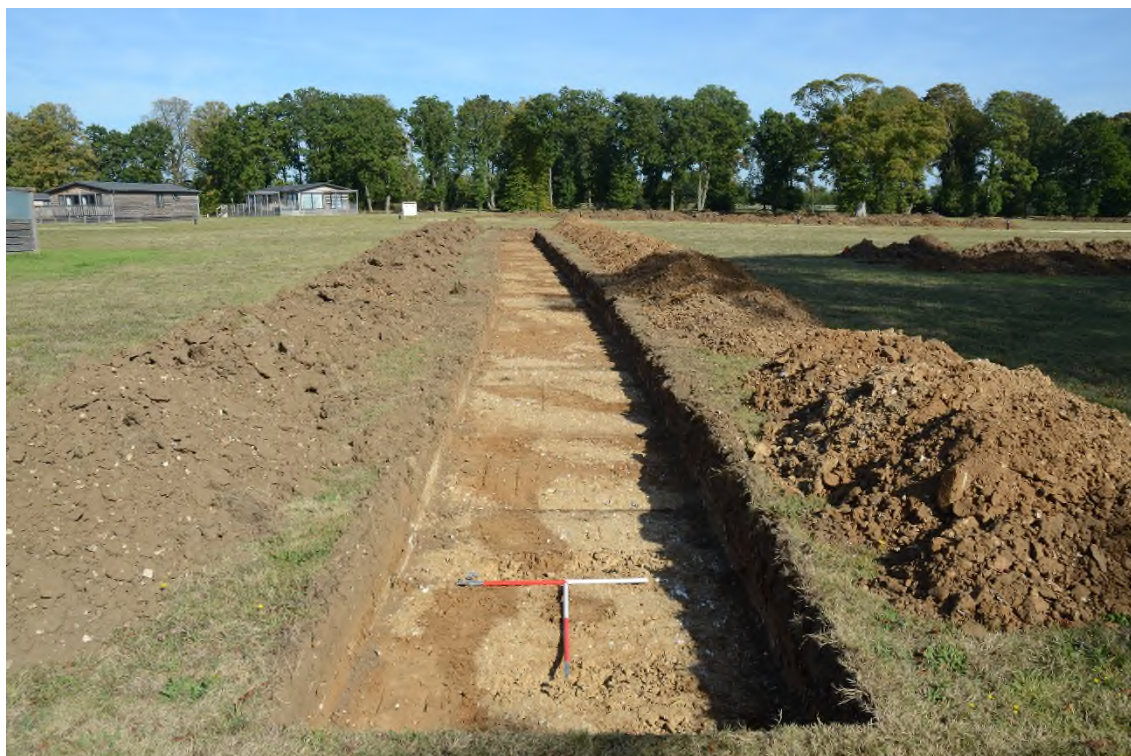
Plate 4: Trench 1, view east
