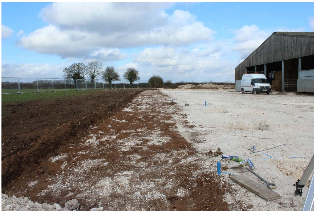
Plate 2. Milking Parlour Building Footings, View North
