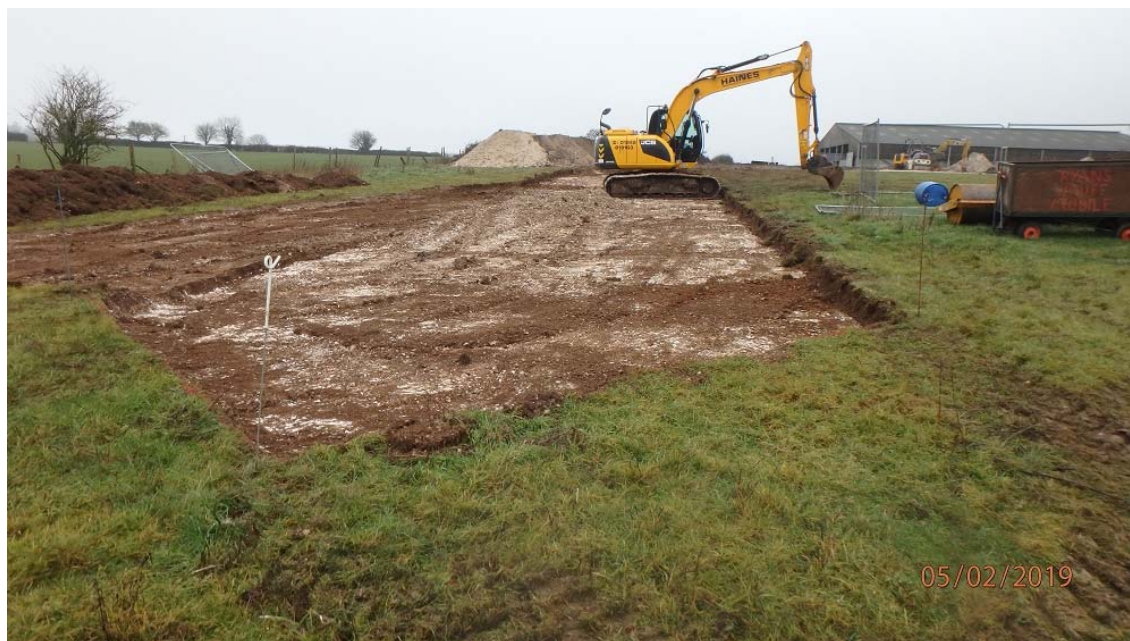
Plate 3. Soak-away Trench, View North
