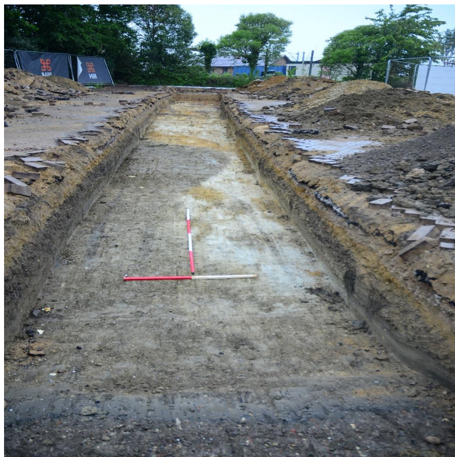
Plate 6: Trench 10 with Pits [1008] and [1010] view west
