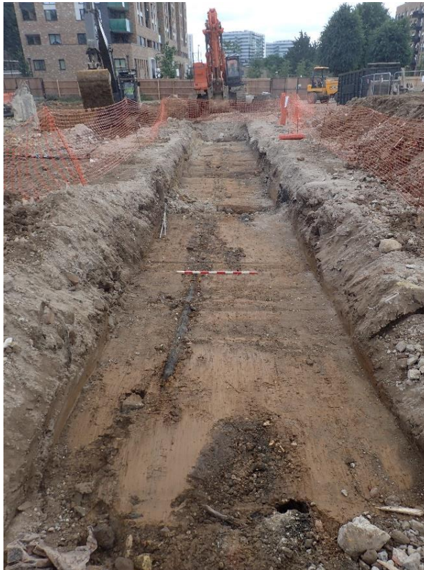
Plate 4: South view of Trench 4 (1m scale).
