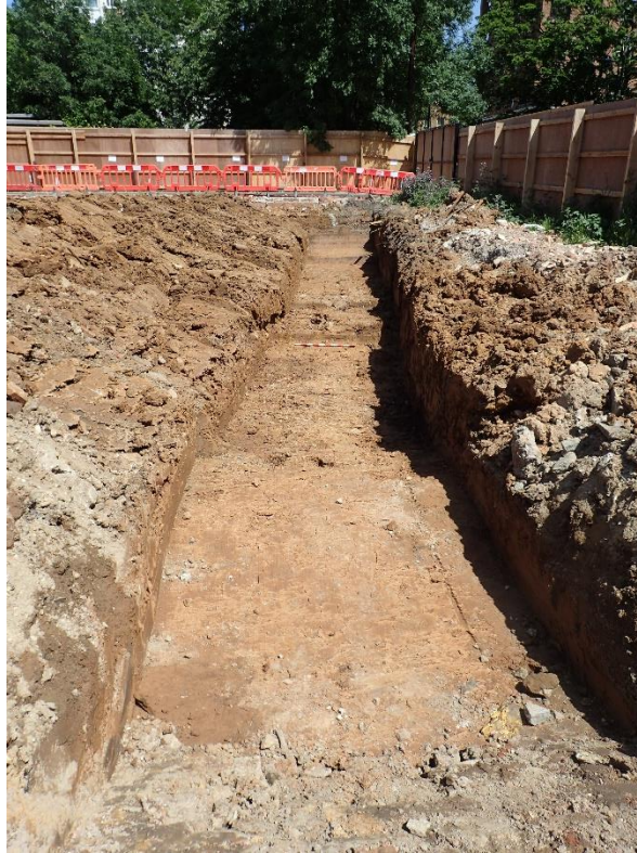
Plate 1: East facing view of Trench 1 (1m scale).
