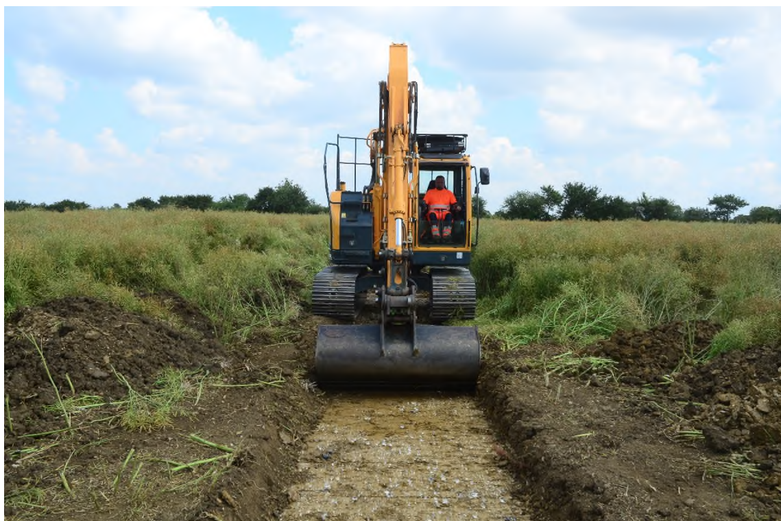
Plate 2: Machining, looking northwest
