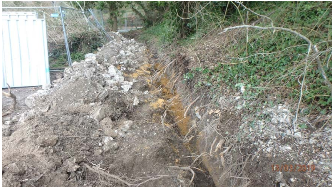
Plate 5 View to the north of service trench
