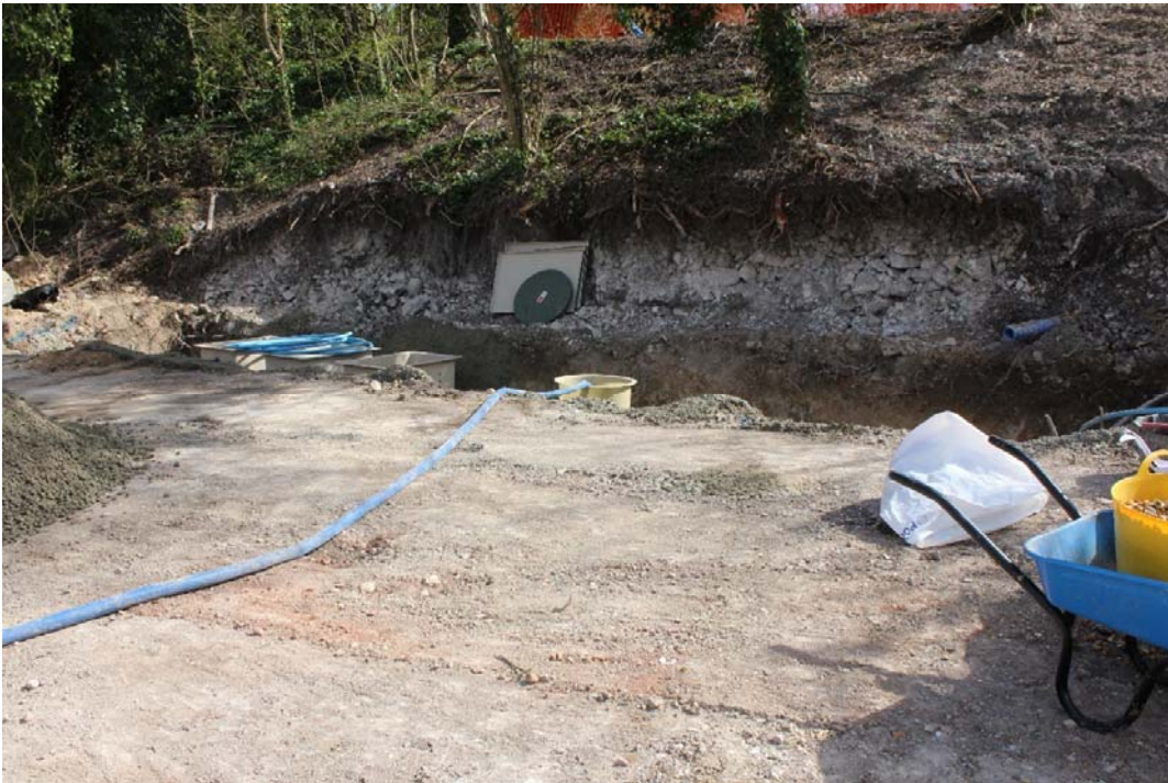
Plate 4 View to the north west section through embankment
