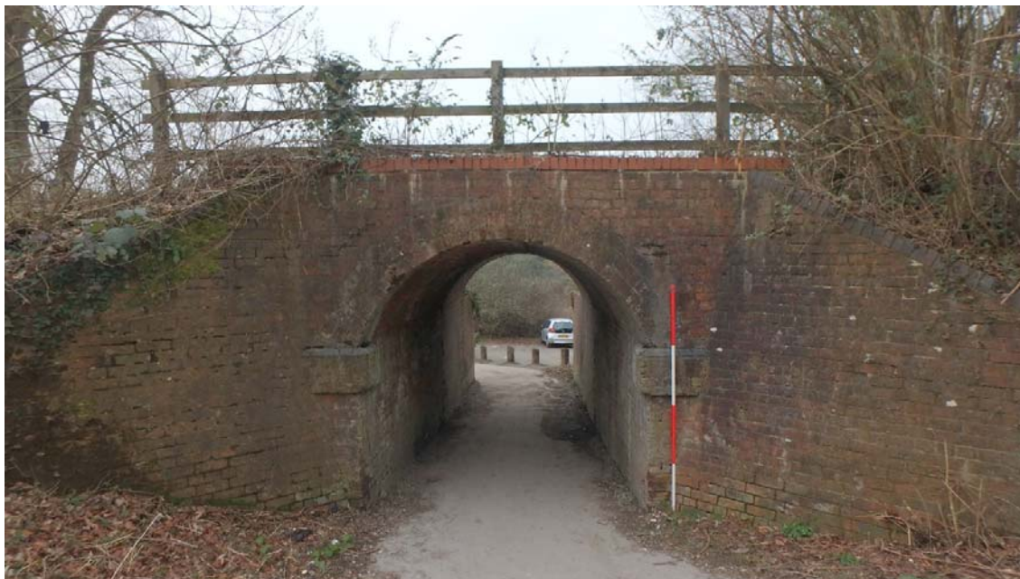
Plate 7 View to the west of 19th century pedestrian railway bridge
