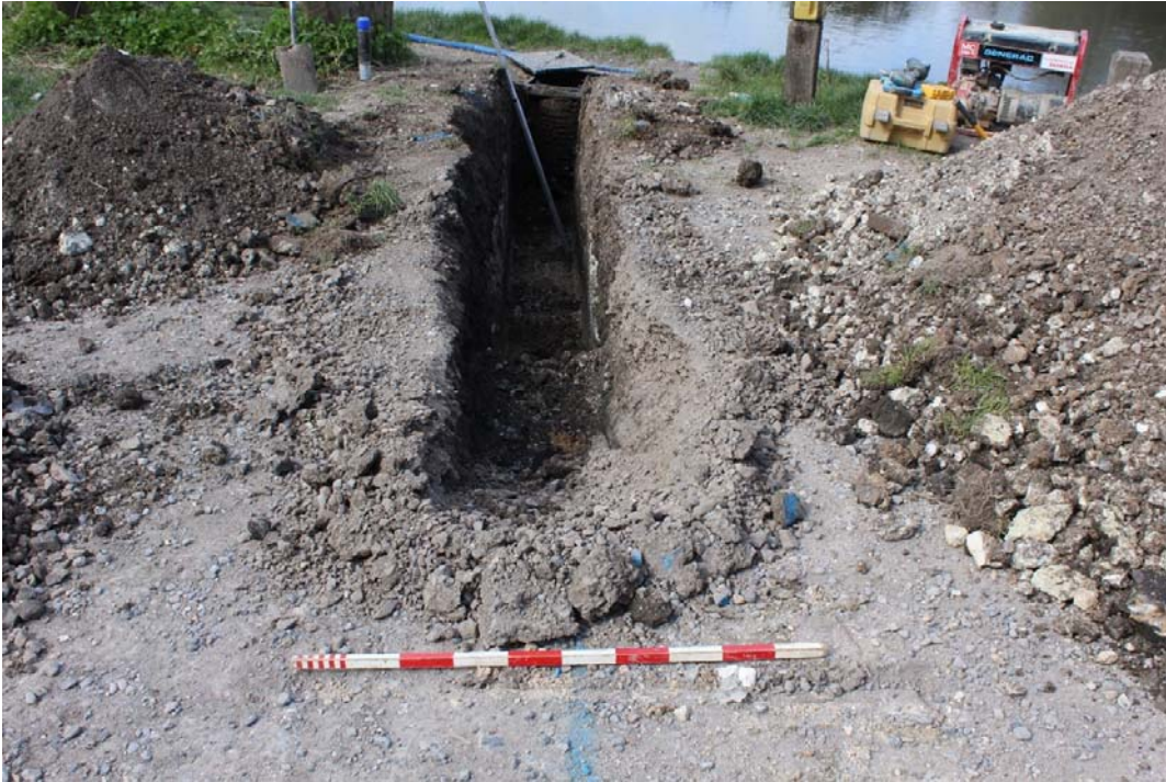
Plate 3 View to the south east of service trench - across car park
