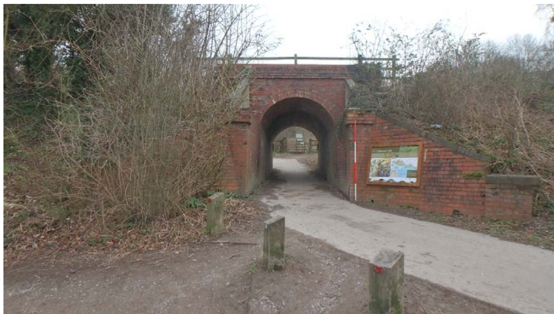
Plate 6 View to the east of 19 th century pedestrian railway bridge
