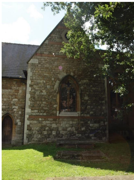
Plate 5: North Porch, looking south
