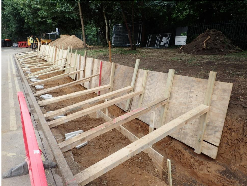
Plate 2: View of bank facing west, post-excavation
