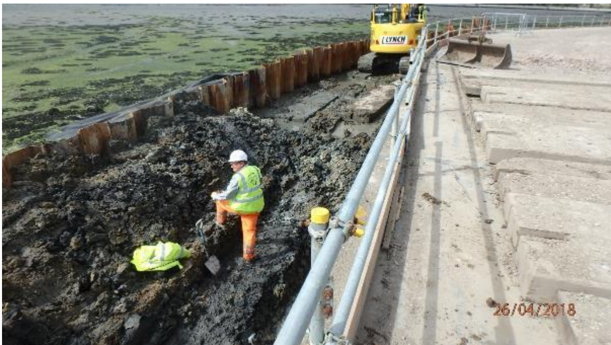
Plate 6. North facing shot of site works, Zone 2.
