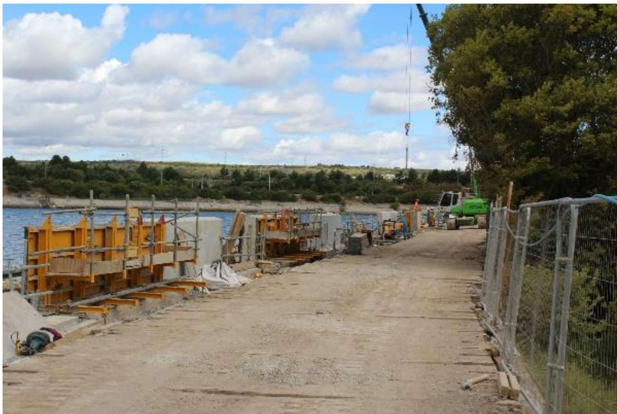
Plate 7. North facing shot of site, Zone 2.
