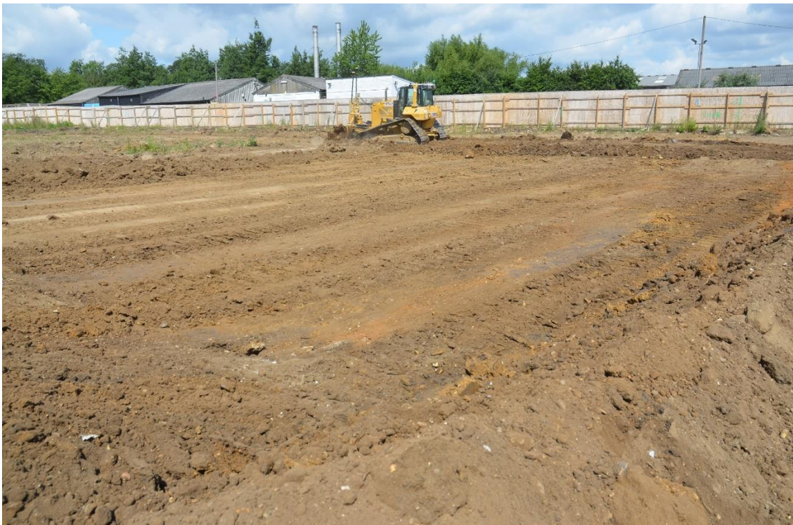
Plate 2: Monitoring Area B, ground reduction, looking north-west.
