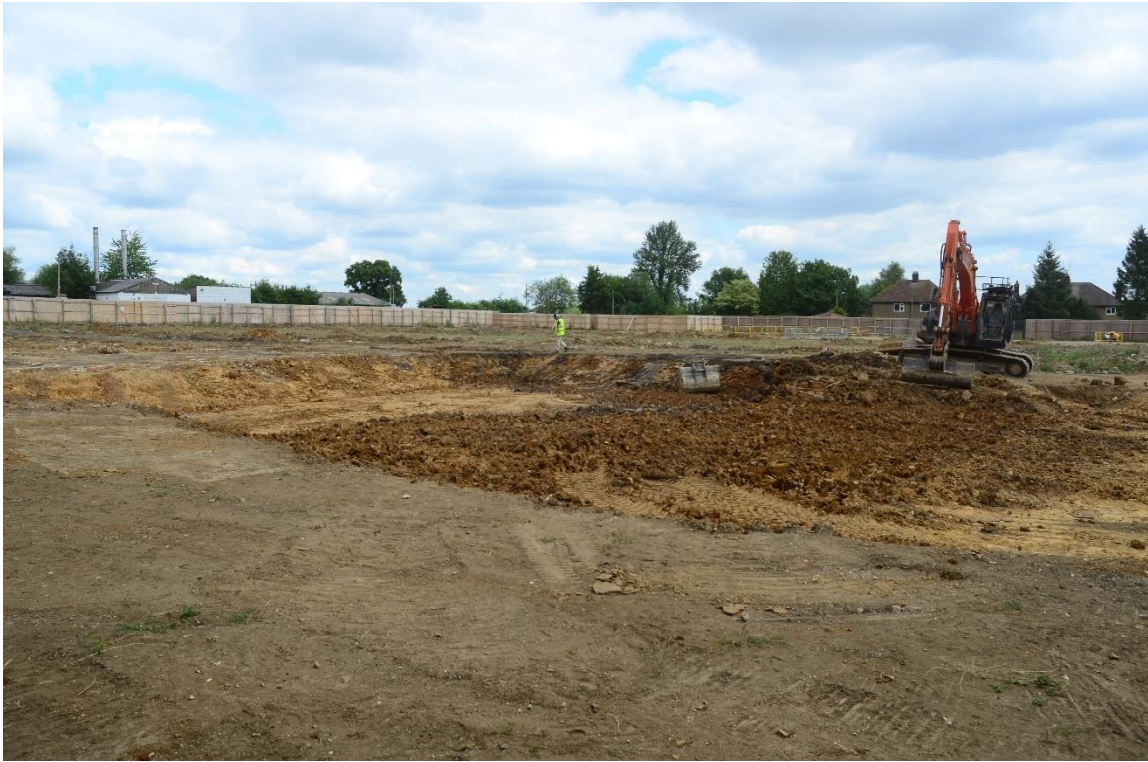
Plate 1: Monitoring Area A during excavation, looking north-east.
