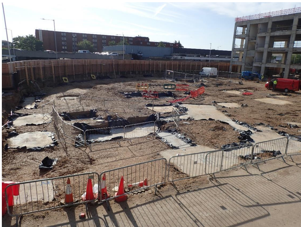
Plate 1: Area 1, looking south-east
