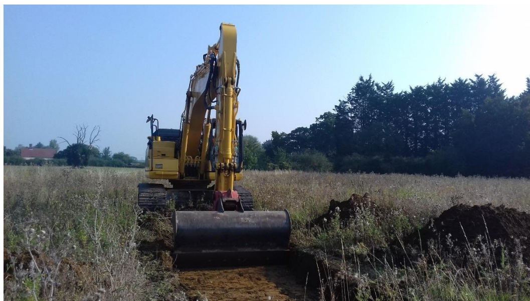
Plate 1: View NE showing Trench 2 and north of site
