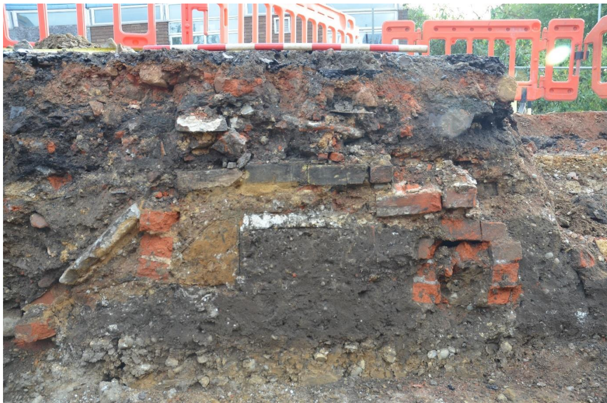
Plate 3: Trench 1, west-facing section showing 1970s demolition (114) and asphalt surface (113) overlying Floor (117), robbed Wall [125], Drain [123] and (beneath) soil Layer (145)
