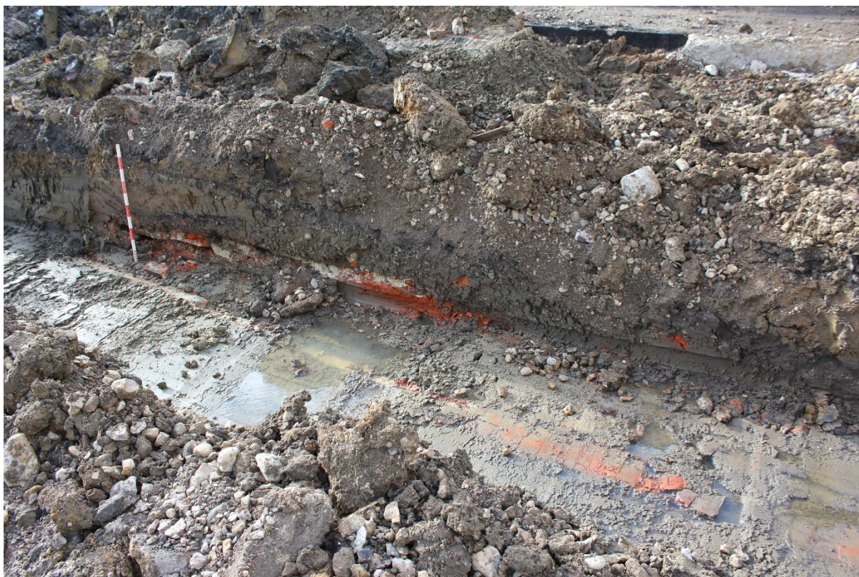
Plate 4 View to the south-east of culvert
