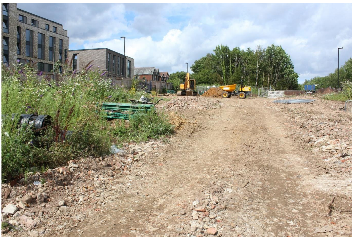
Plate 6 View to the north of proposed watching brief area (former basement)
