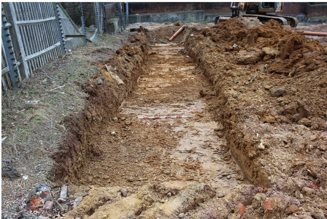
Plate 1 View to the east of Trench 1
