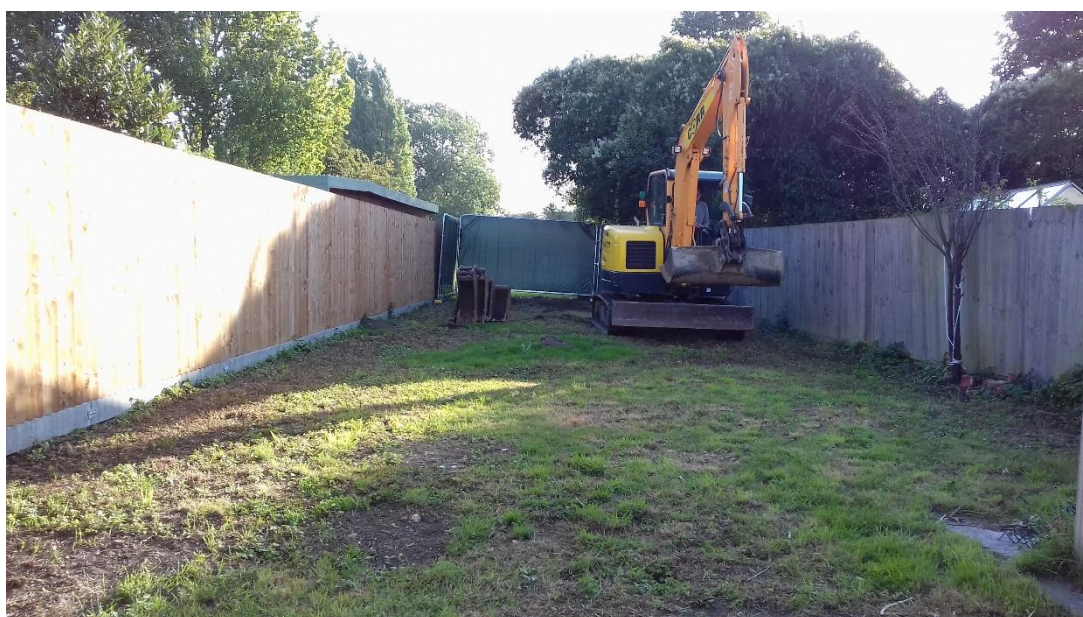
Plate 2: Pre-excitation. View NE, site with 6 tonne excavator
