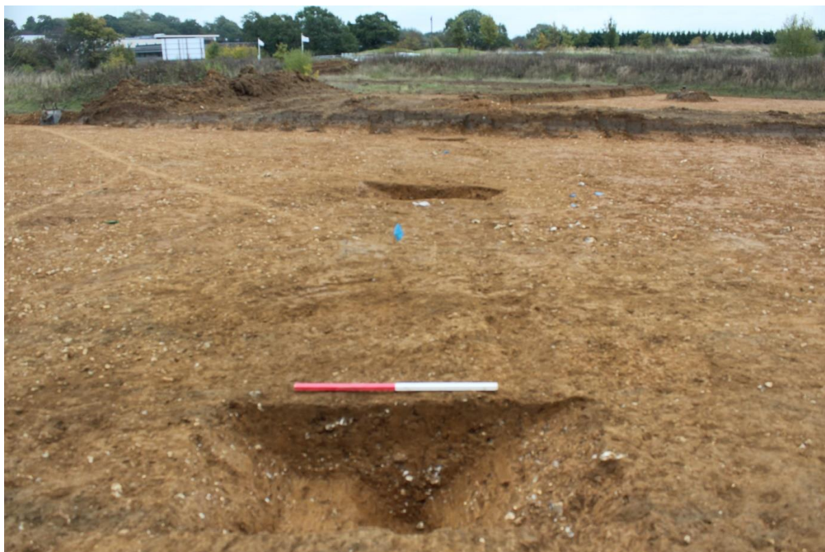
Plate 4: Ditches 5 and 6, looking south-west
