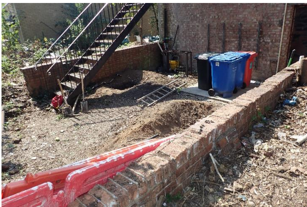
Plate 1: The site, looking north-east
