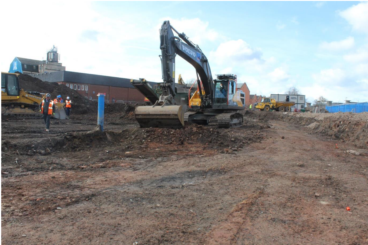
Plate 1: Working shot, looking west
