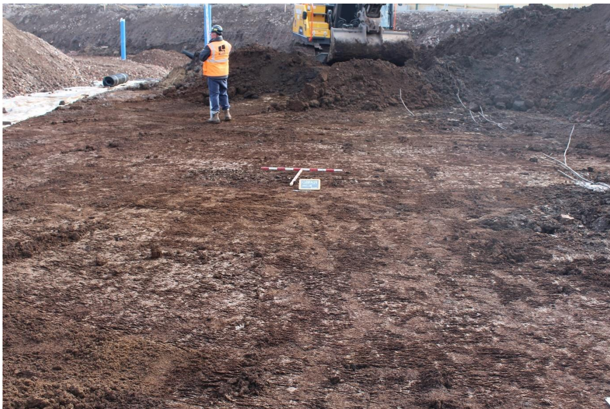
Plate 6: Base of excavation at southern end of area, looking east
