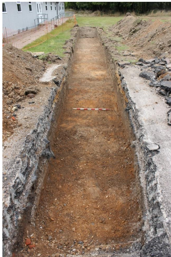
Plate 4: Trench 3 facing west, 1m scale
