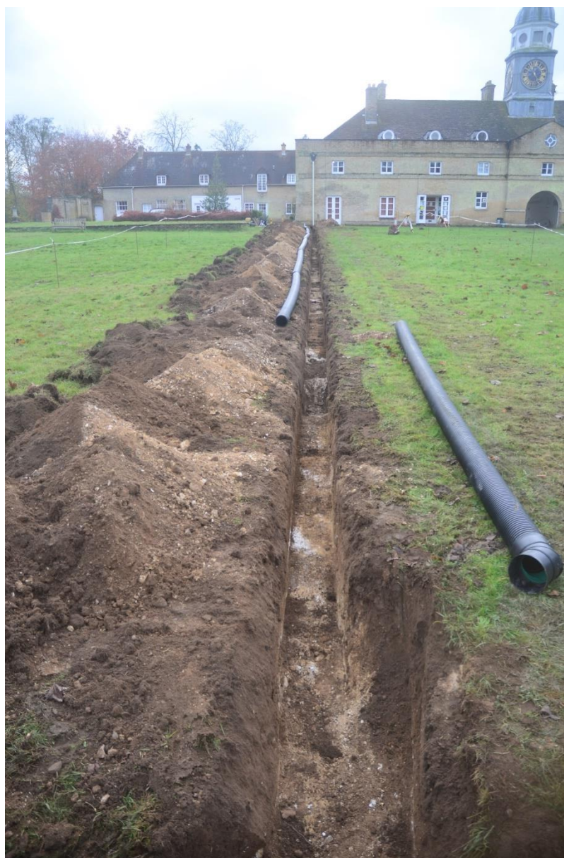
Plate 6: Pipe trench, view south
