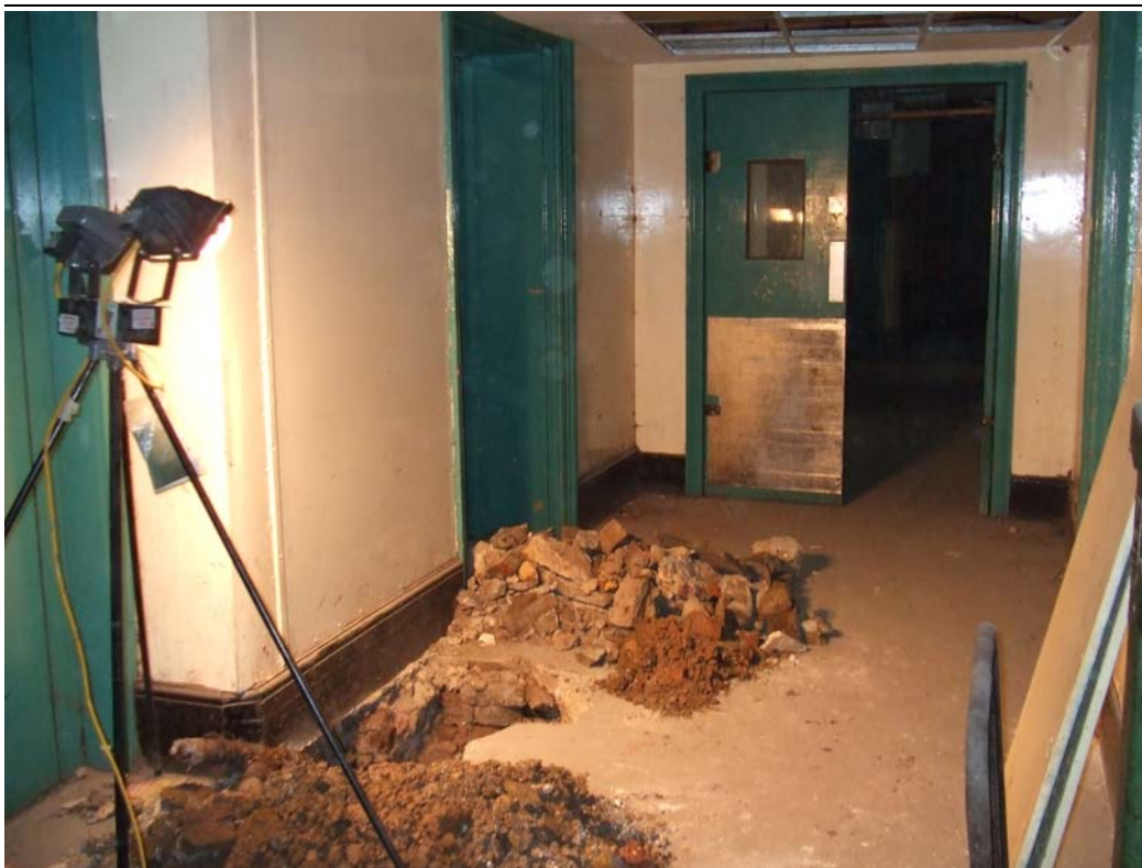
Plate 3 Trial Pit 21, showing general site conditions
