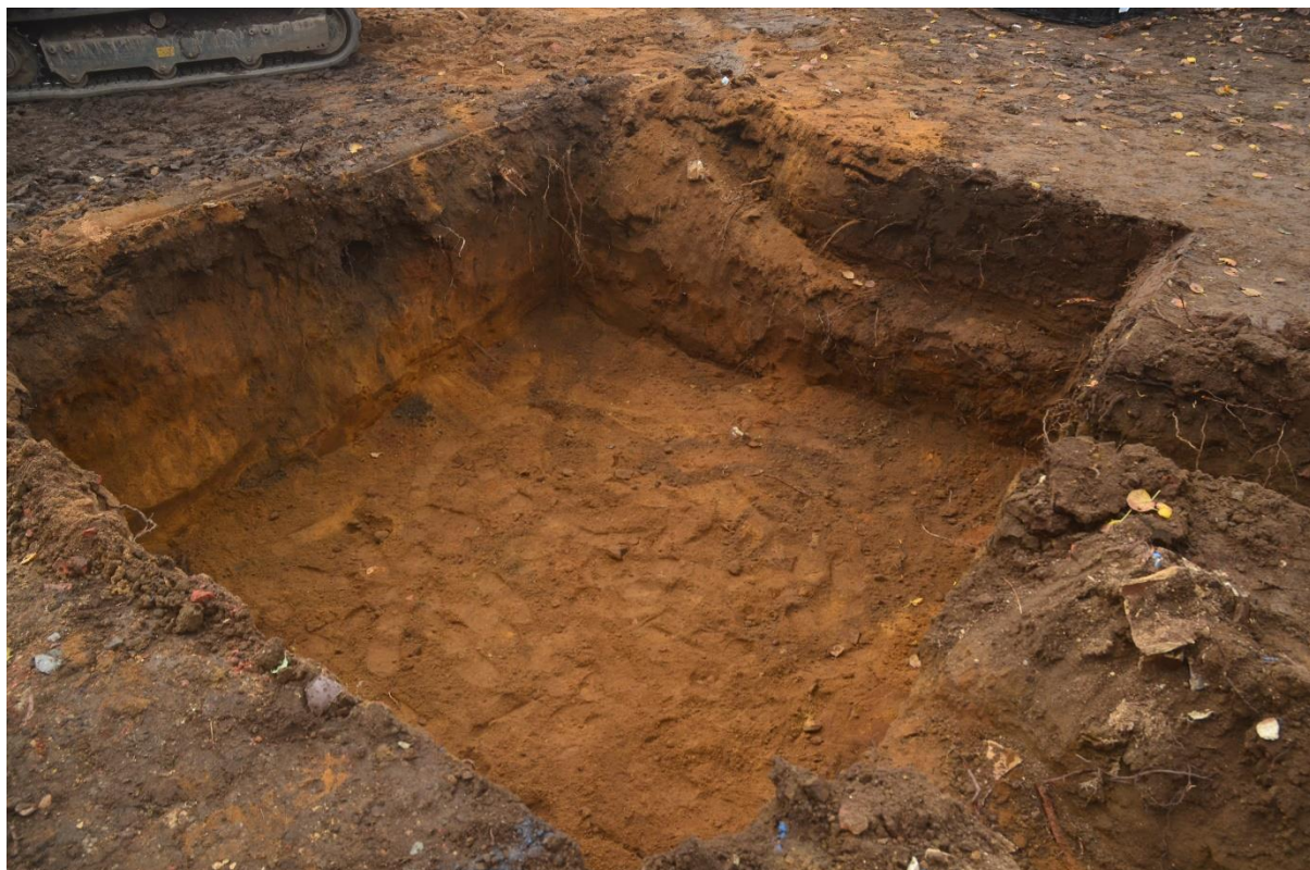
Plate 7: The soakaway, view south-west
