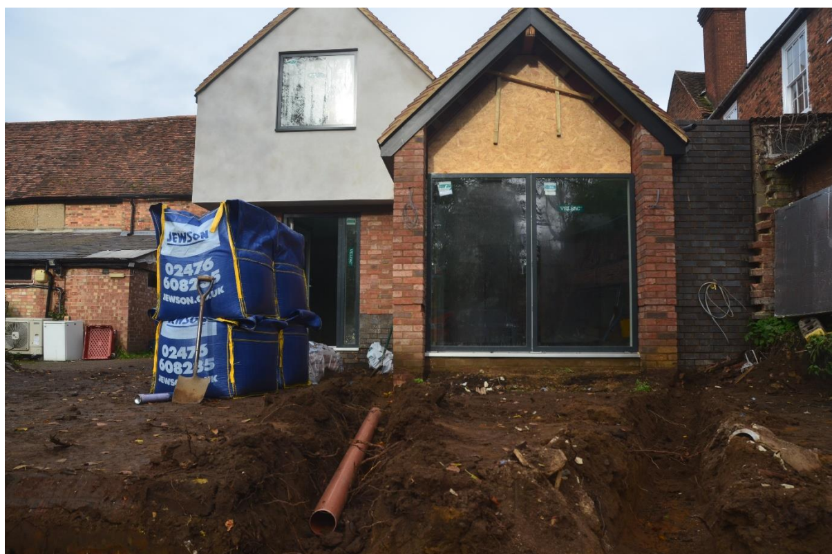
Plate 6: The completed extension, view north
