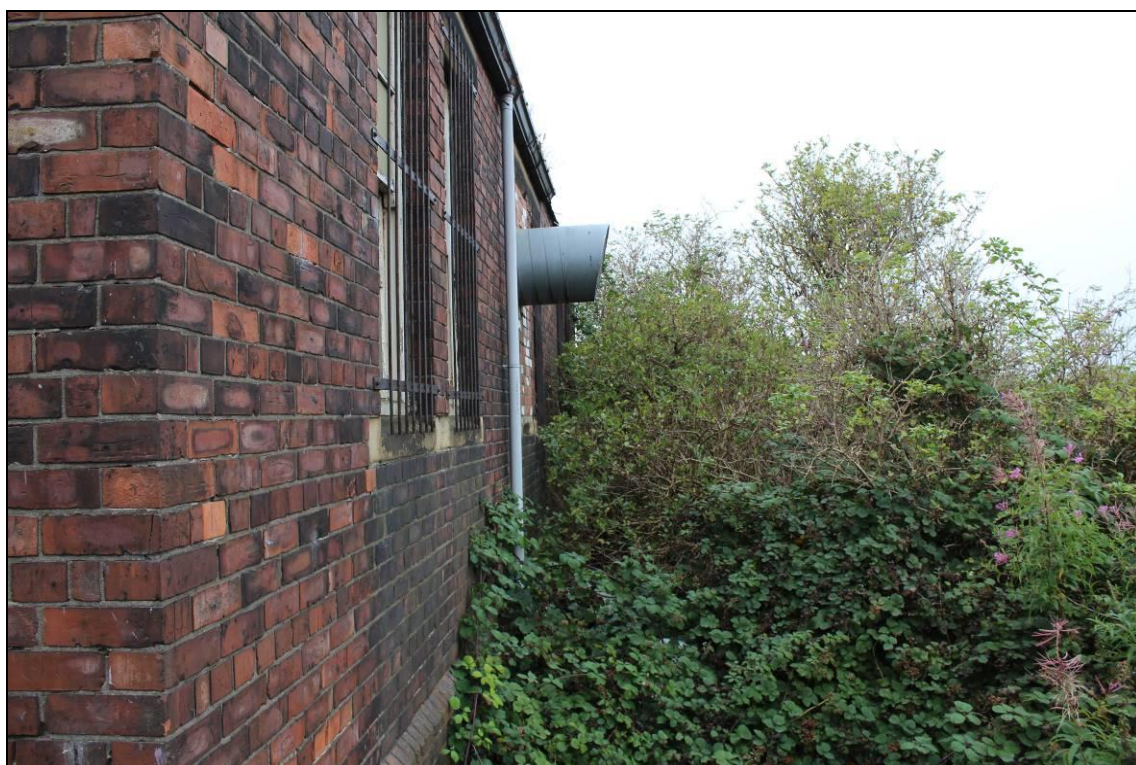
Plate 18: Exterior of Room 4: view west
