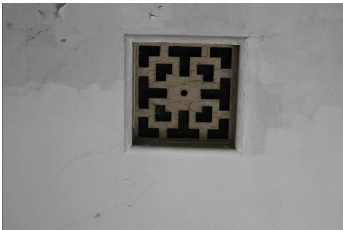
Plate 57: Roof 3a, decorative loft hatch
