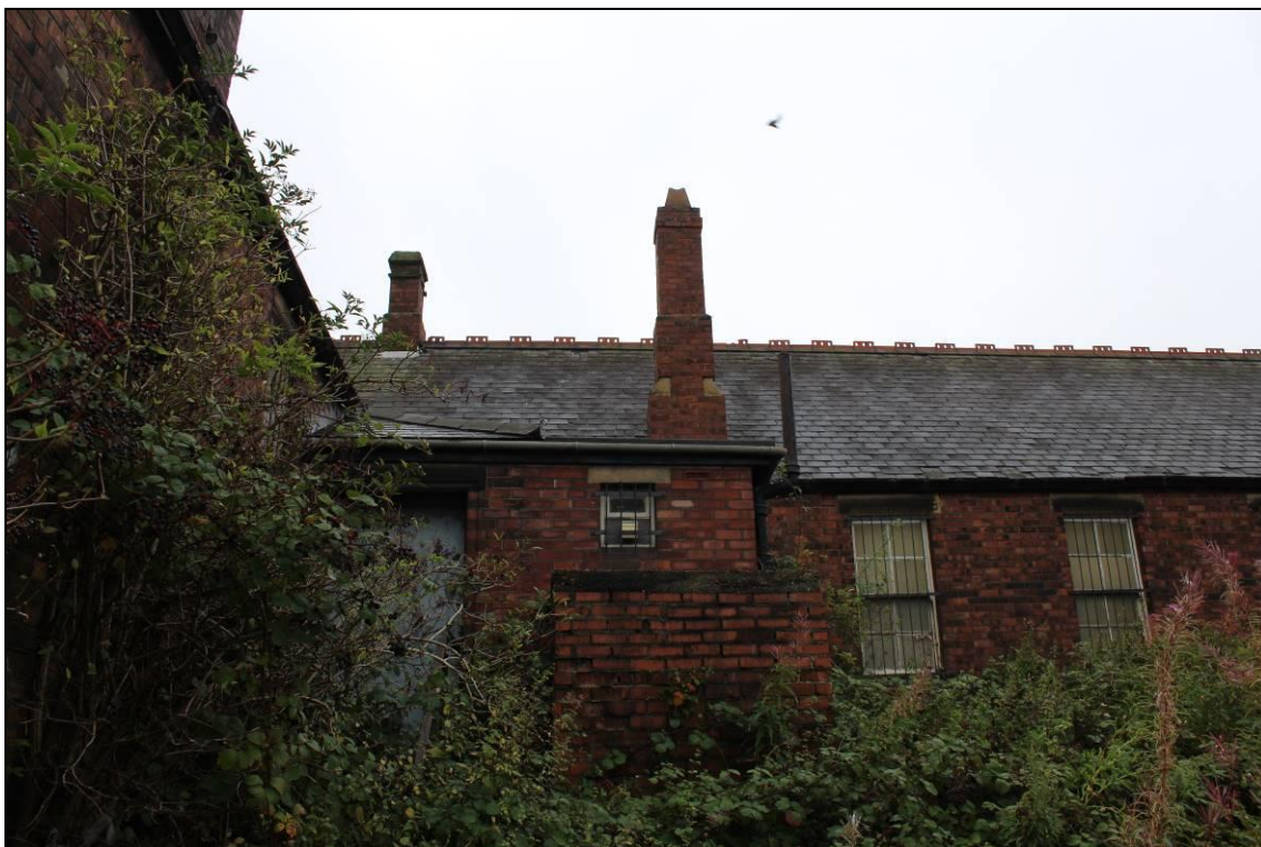
Plate 16: Northern exterior of Room 2: view south
