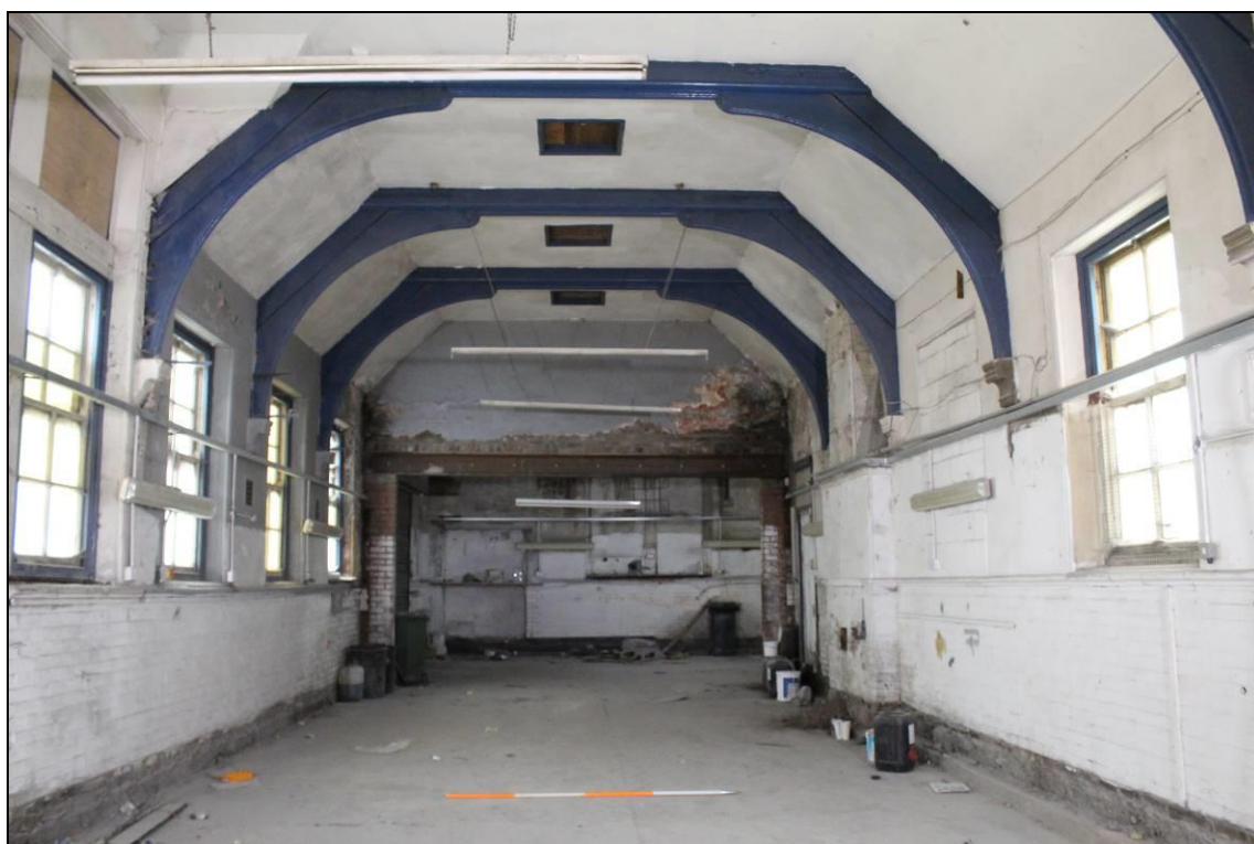
Plate 58: Room 3b, view west, scale: 2m
