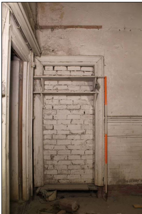
Plate 46: Room 3a, bricked up doorway: view east, scale: 2m
