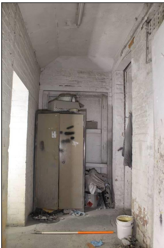
Plate 37: Room 2a: view north, scale: 1m
