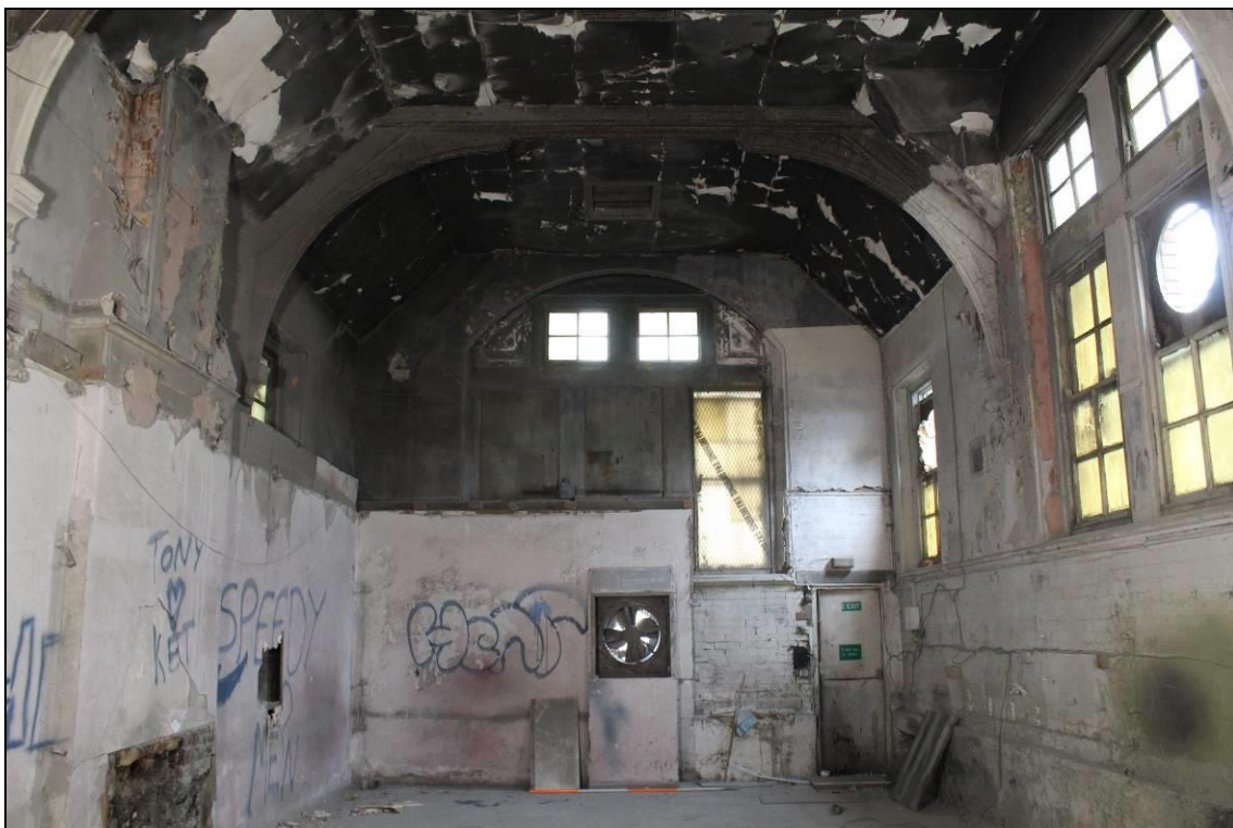
Plate 31: Room 1b, north wall: view north, scale: 2m
