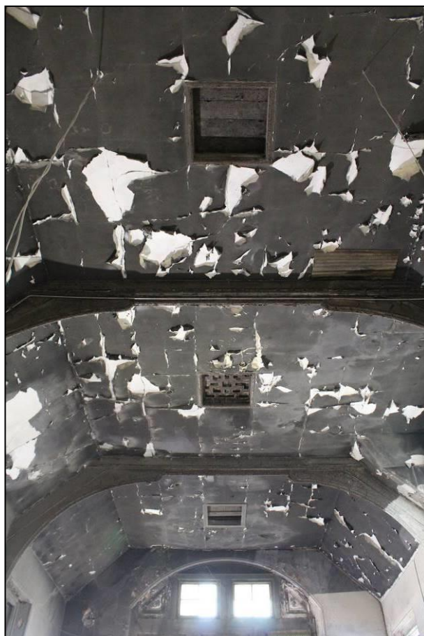
Plate 36: Room 1b, timber roof trusses and loft hatches: view north
