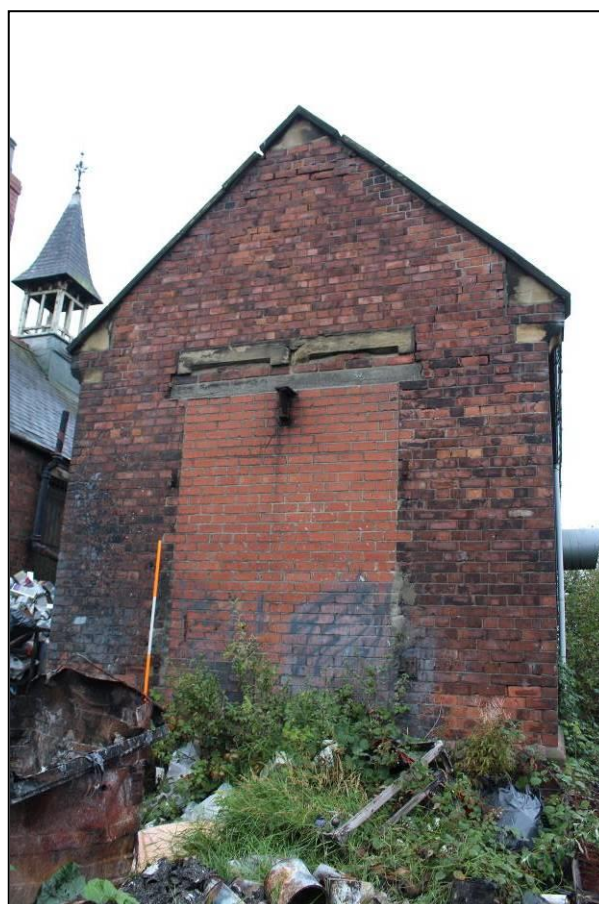
Plate 20: Exterior of Room 4 showing bricked up 20th century entrance: view southwest, scale: 2m
