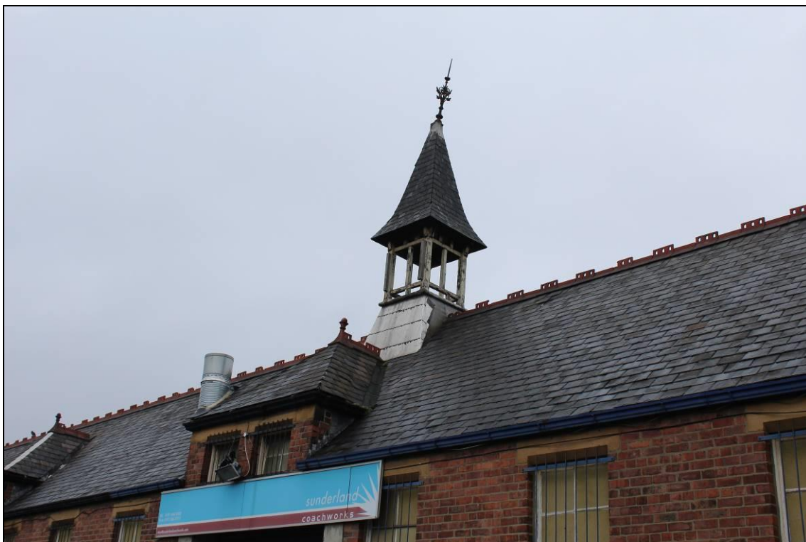
Plate 5: Bellcote: view northwest
