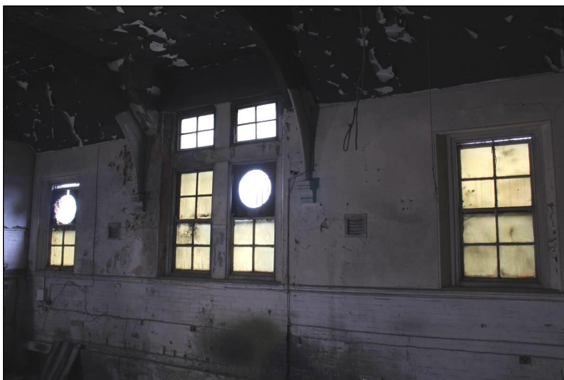
Plate 30: Room 1b, east wall: view northeast
