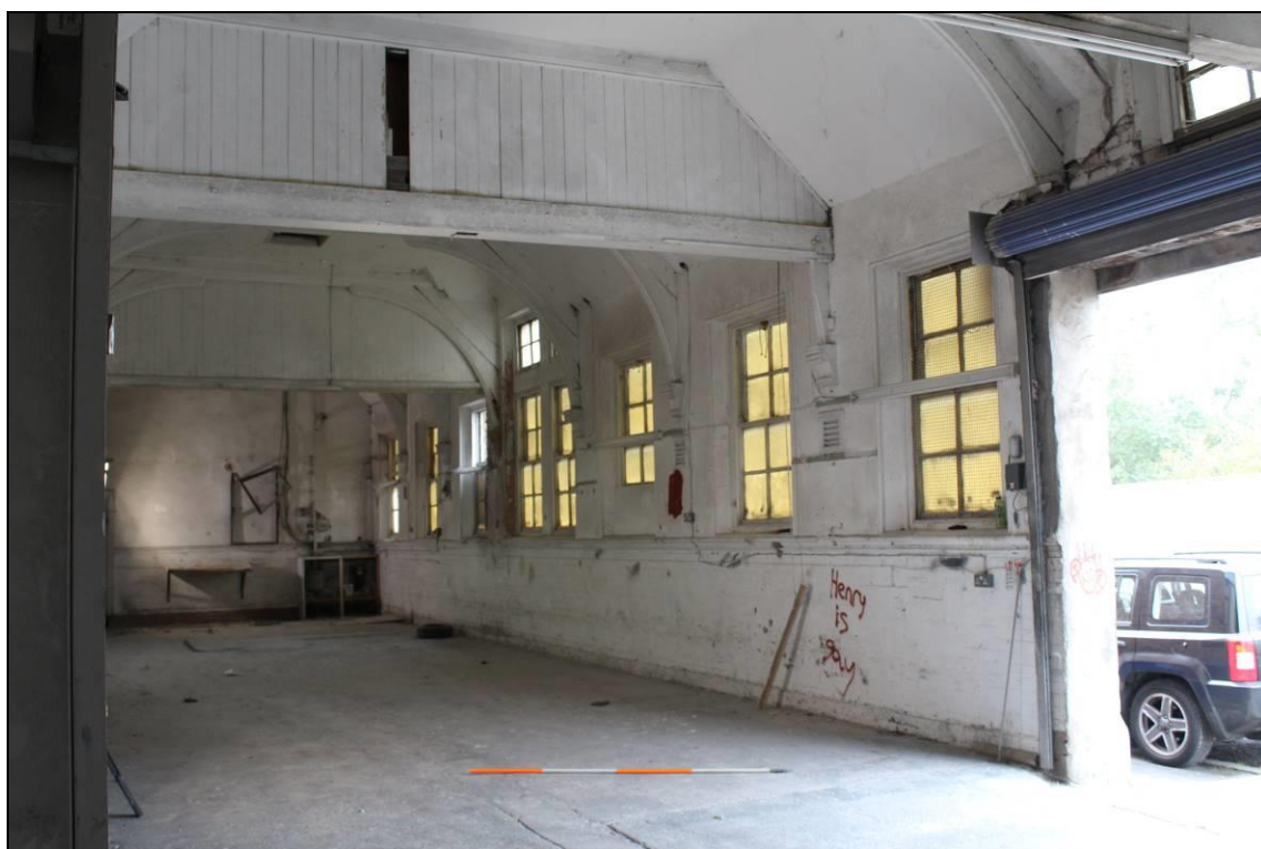
Plate 47: Room 3a: view southeast, scale: 2m
