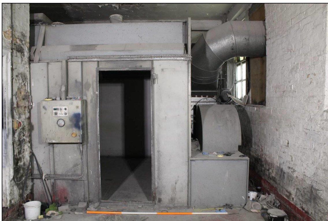
Plate 68: Room 4a, spraying dock: view west, scale: 2m
