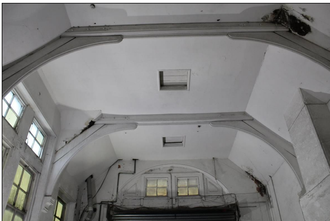
Plate 26: Room 1a, timber roof trusses and loft hatches: view south
