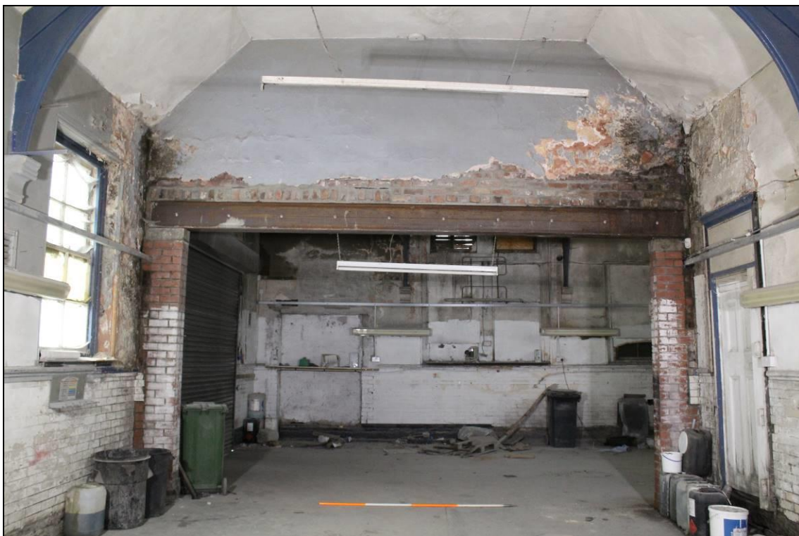
Plate 63: Room 3b: view west, scale: 2m
