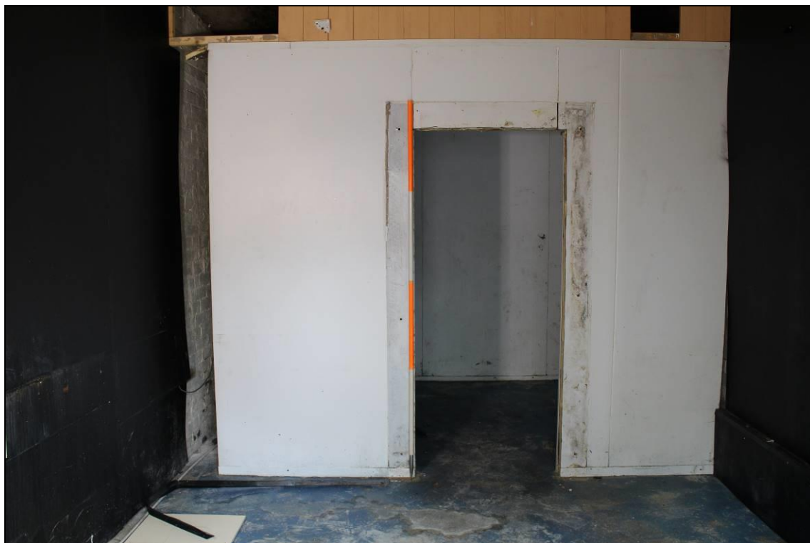
Plate 83: Room 7a & 7b: view north, scale: 2m
