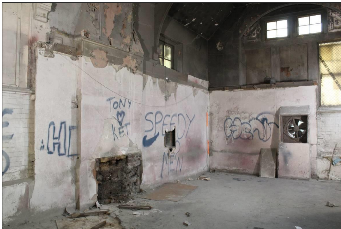
Plate 29: Room 1b, modern plasterboard obscuring original windows and chimney breast: view northwest, scale: 2m
