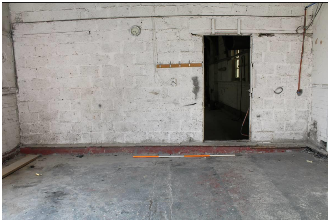
Plate 55: Room 3a & 3b, partition: view west, scale: 2m
