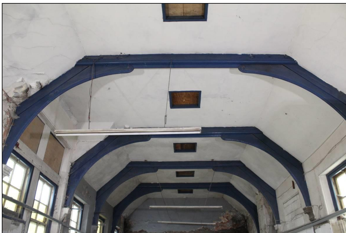
Plate 62: Room 3b, Timber roof trusses and loft hatches: view west
