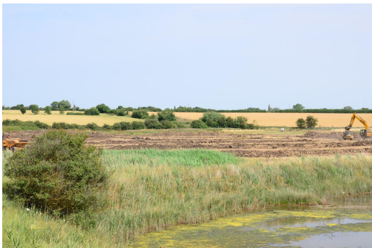
Plate 4: Stripping of Borrow Pit
