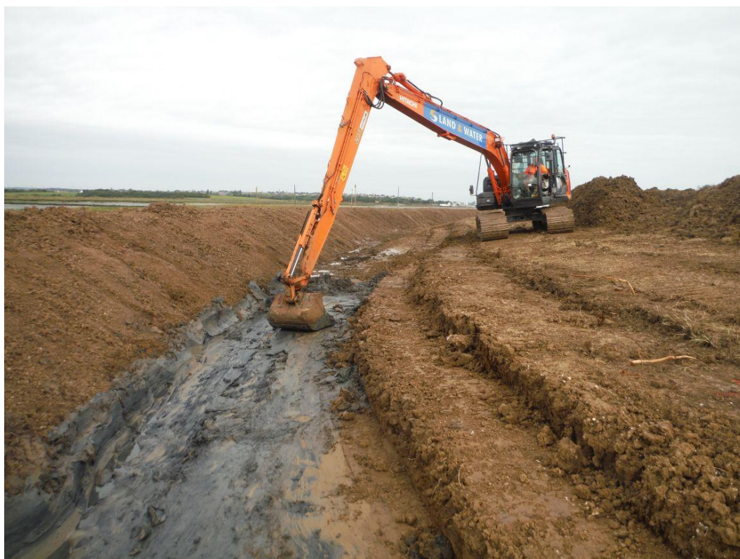
Plate 3: Landscaping of borrow ditch and landward bank. Natural clay visible at base of ditch
