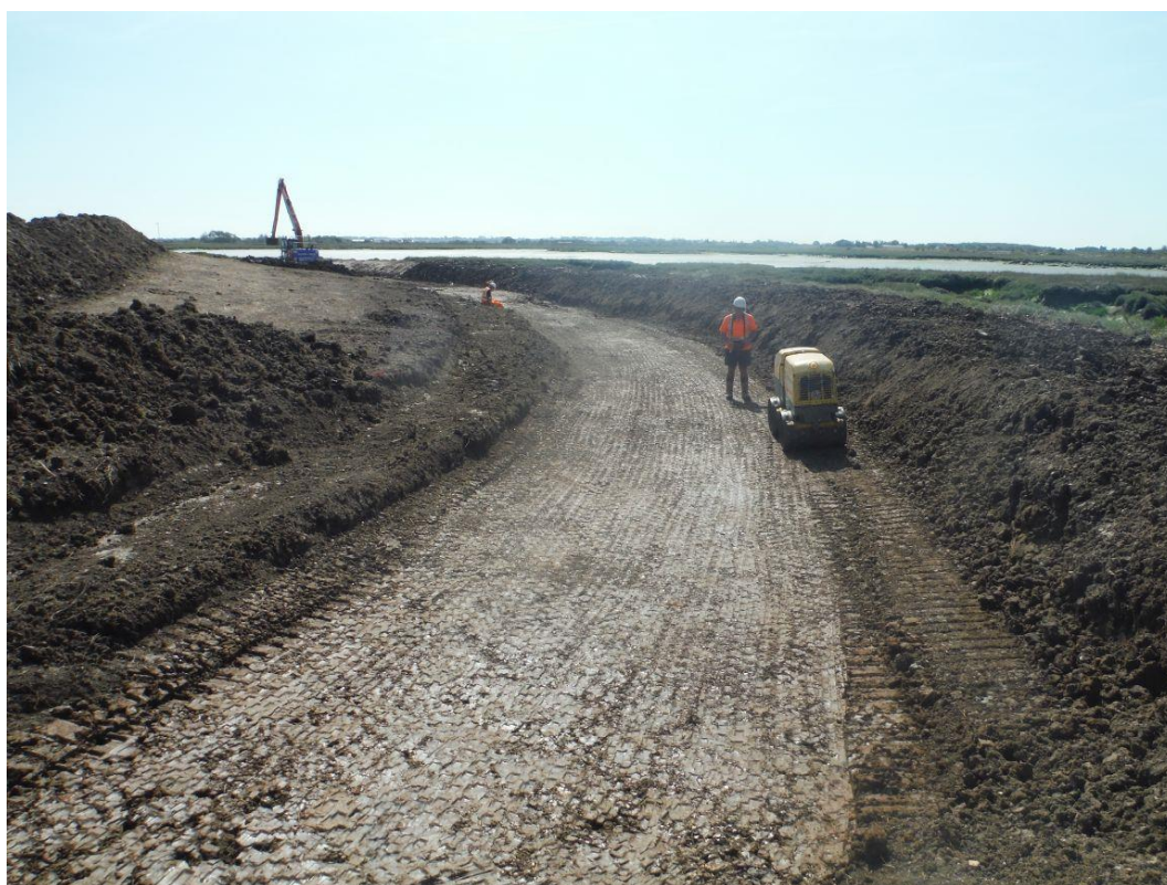
Plate 4: Infilled borrow ditch
