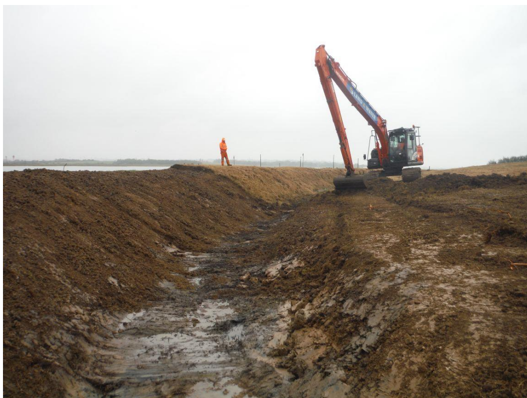
Plate 2: Lowering of sea bank and clearing out of borrow ditch
