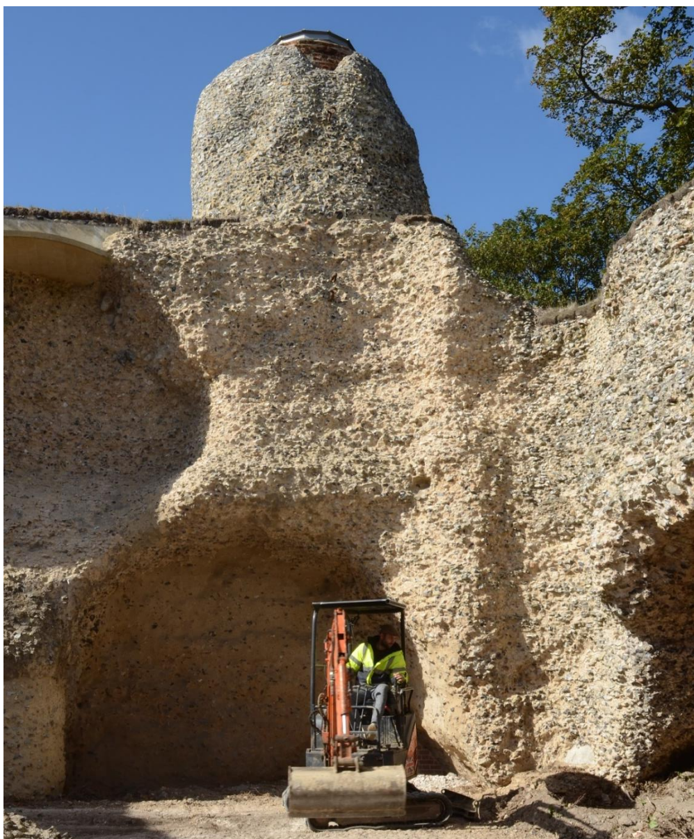
Plate 3: view south, levelling the ground inside the keep
