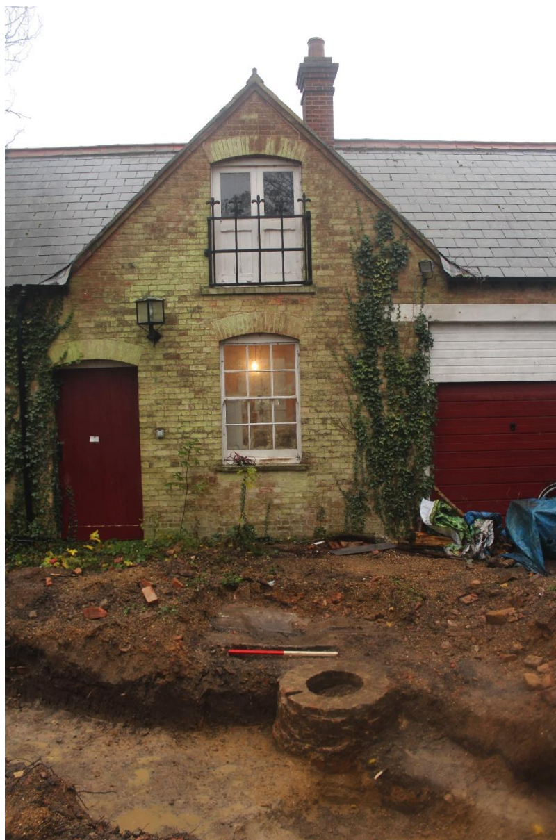
Plate 4: Soakaway (124) with coach house, view south
