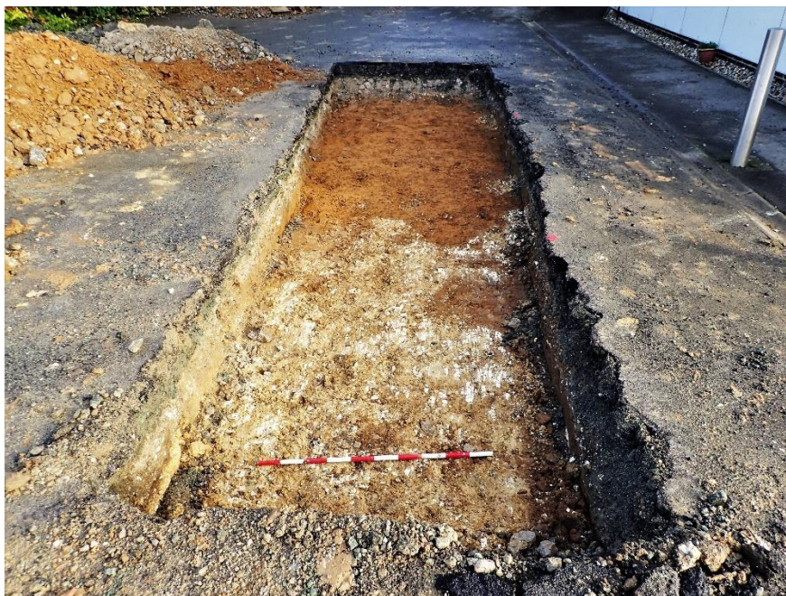
Plate 1: Trench 1, view to the north-east, scale 1m. Chalk bedrock [9] in foreground.
