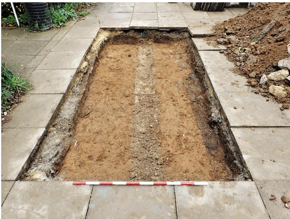
Plate 5: Test Pit 2, view to north-east, scale 1m.
