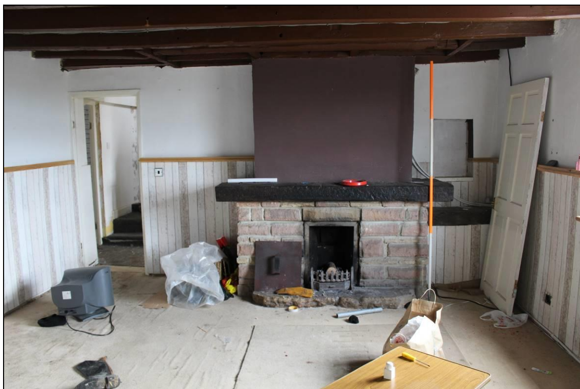
Plate 13: Building A: Room A1.7: view east 2m scale
