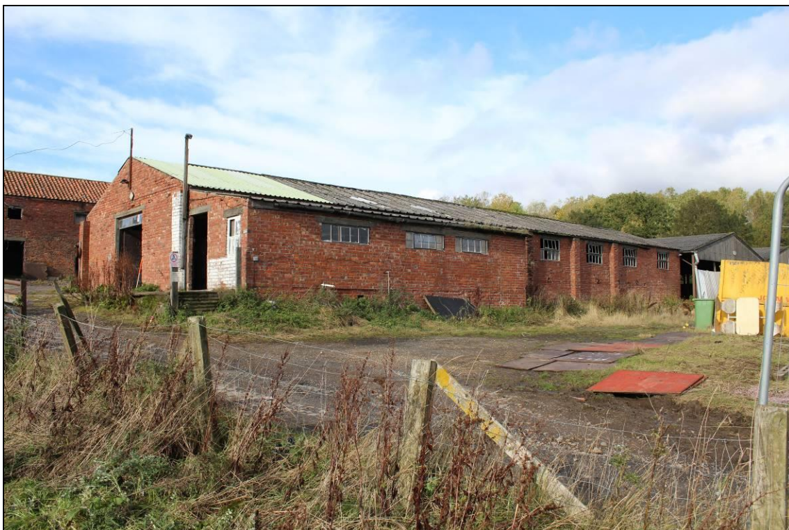
Plate 58: Building E: stable block, view northwest, 2m scale
