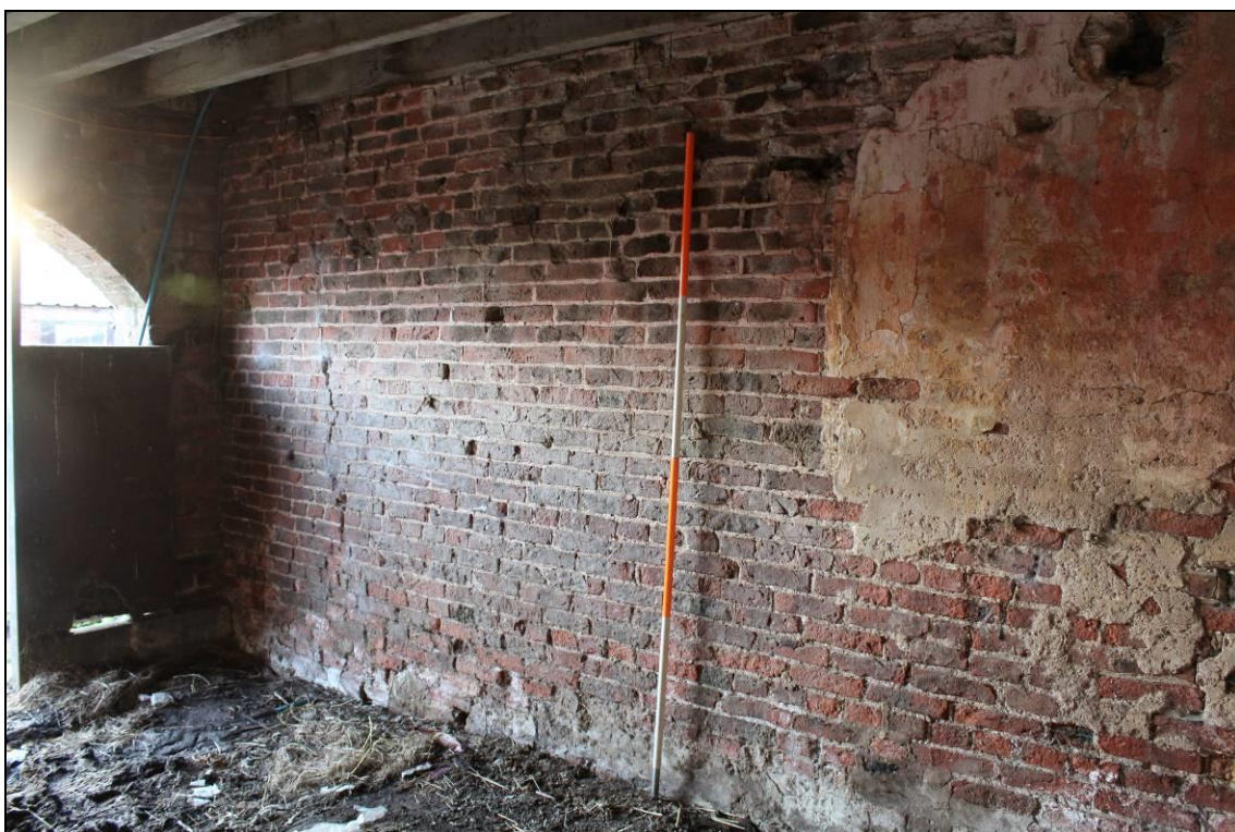
Plate 43: Northern elevation of Building C1: view southeast, 2m scale
