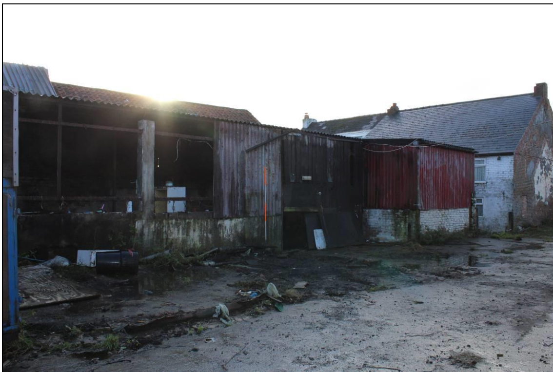
Plate 52: Building C4, west facing elevation: view southeast, 2m scale
