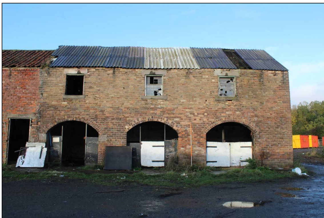
Plate 46: Building C2, hemmel/shelter shed with hay loft above: view west, 2m scale 2m
