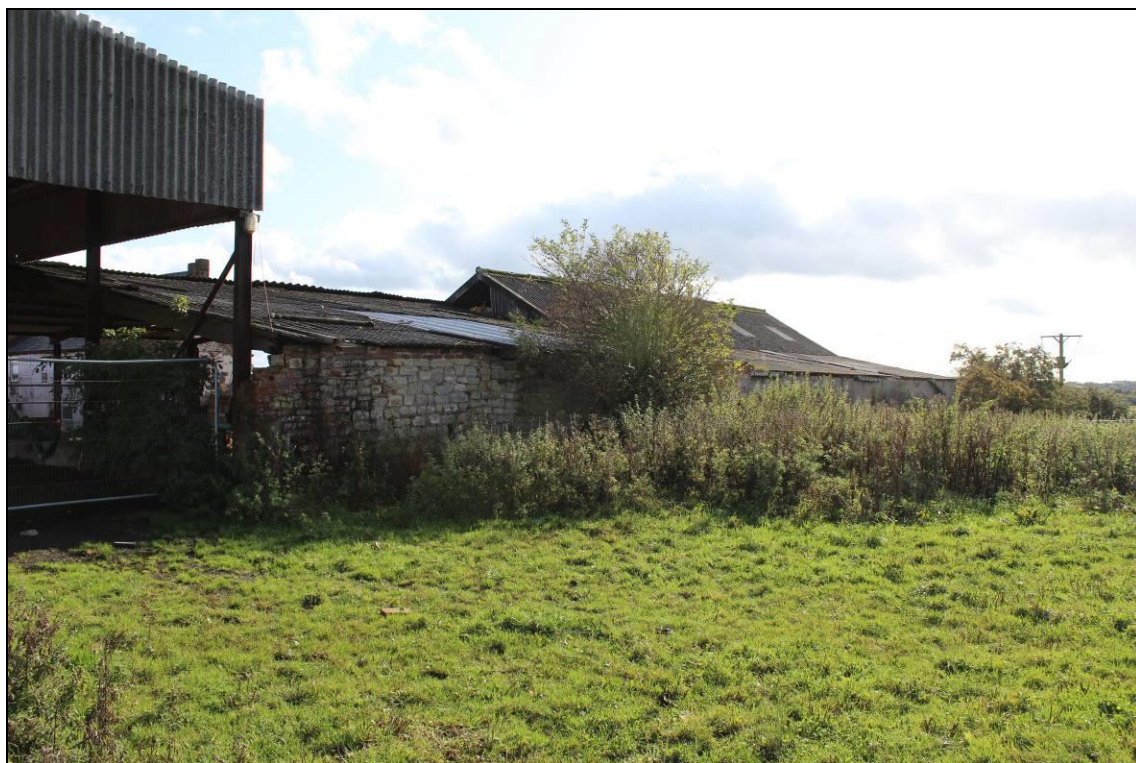
Plate 37: Western wall of Building B2 and B3: view southeast
