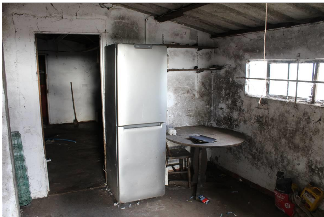
Plate 63: Building E: Room on eastern side: view northeast
