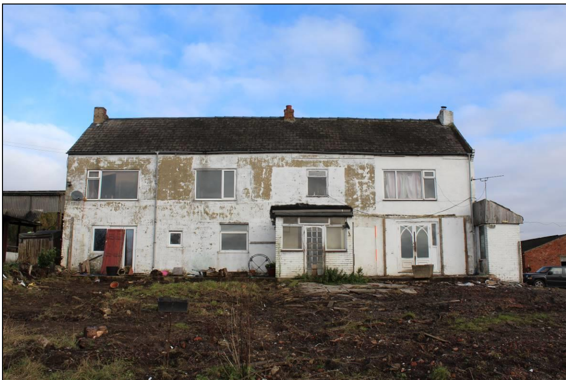
Plate 5: Building A: Farmhouse: view north, 2m scale
