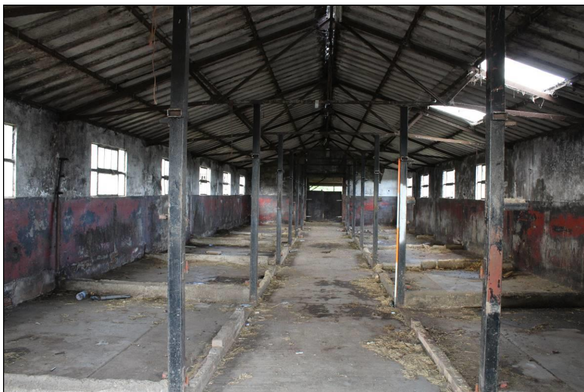
Plate 61: Building E: interior stable block: view north, 2m scale
