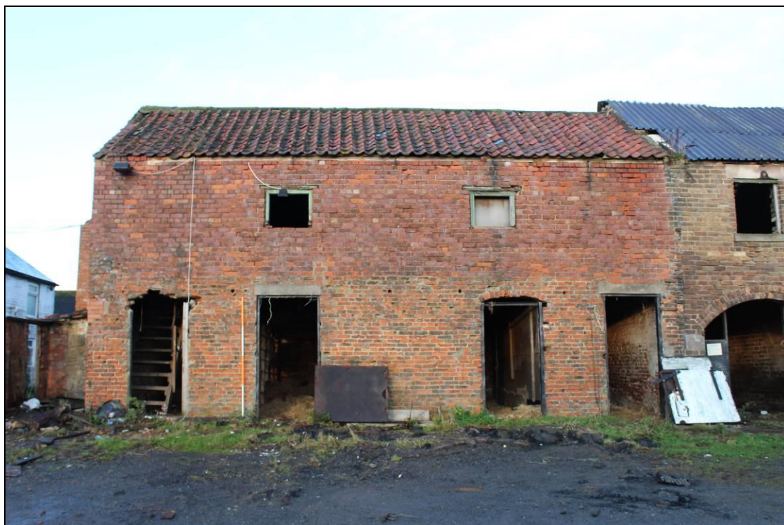
Plate 41: Building C1: stable block with hay loft above. Note brick scar and use of different bricks just above lintels of each doorway: view west, 2m scale
