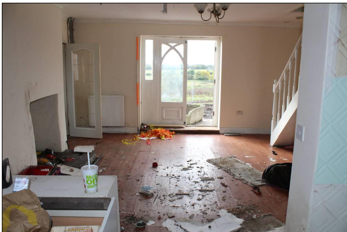
Plate 15: Building A: Room A1.9: view south, 2m scale
