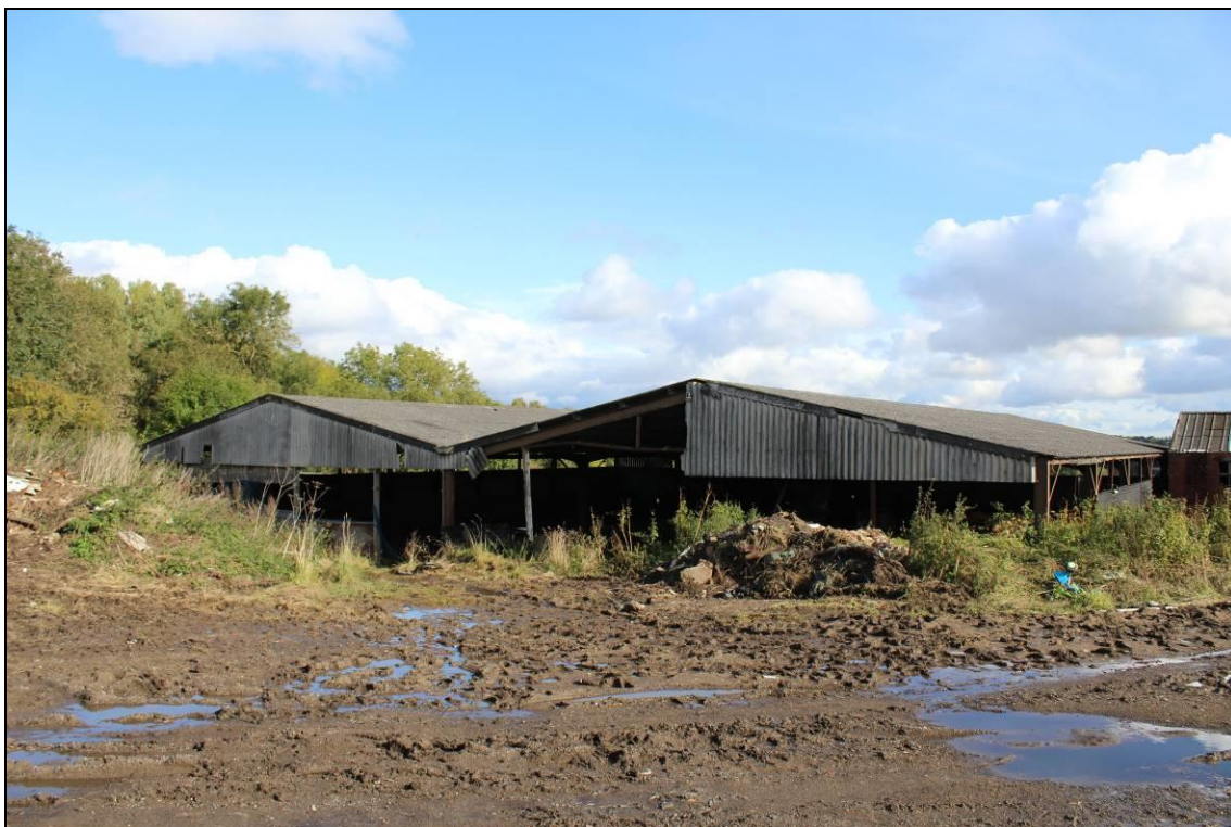
Plate 57: Building D: steel portal frame shed, view northeast
