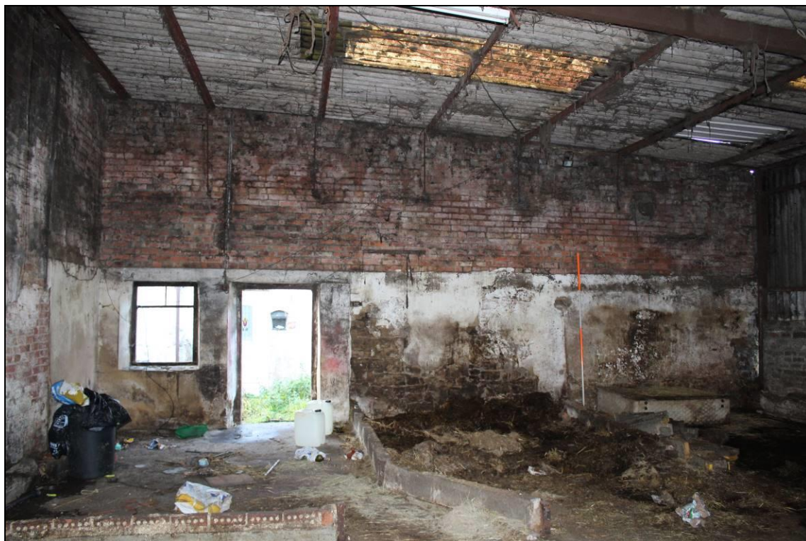
Plate 56: Building C4, internal, southern exterior wall: view south, 2m scale
