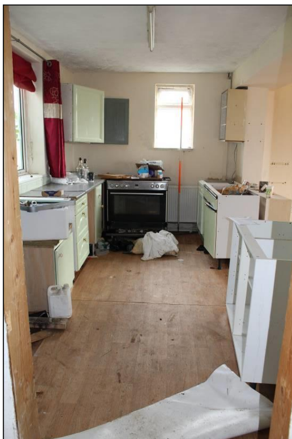
Plate 17: Building A: Room A1.10: view east, 2m scale
