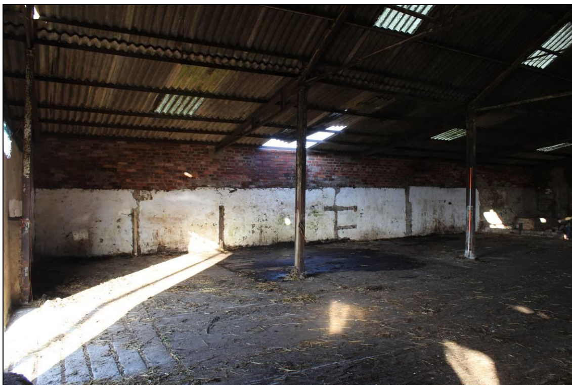
Plate 36: Building B2: interior, western wall, 2m scale
