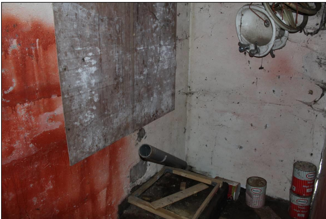
Plate 65: Building E: storage room: view northeast
