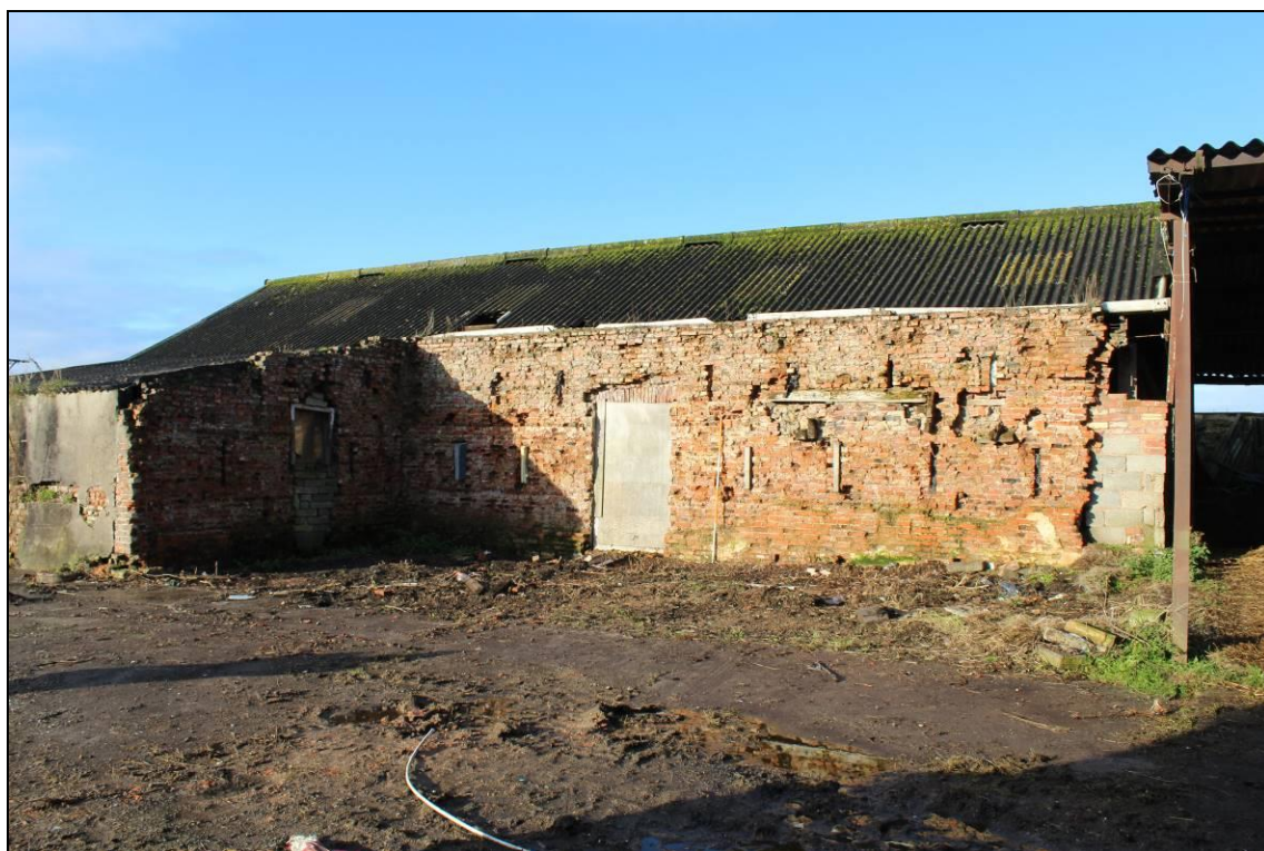
Plate 30: Building B1: view southwest, 2m scale
