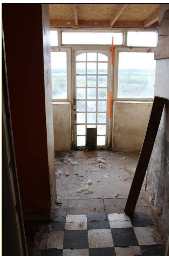
Plate 12: Building A: Room A1.6: view south, 2m scale
