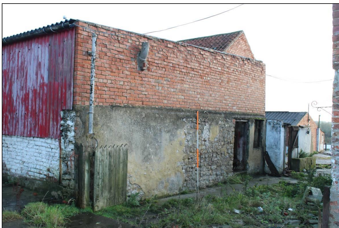
Plate 54: Building C4, south facing elevation (note original sandstone building fabric on lower courses): view northwest, 2m scale
