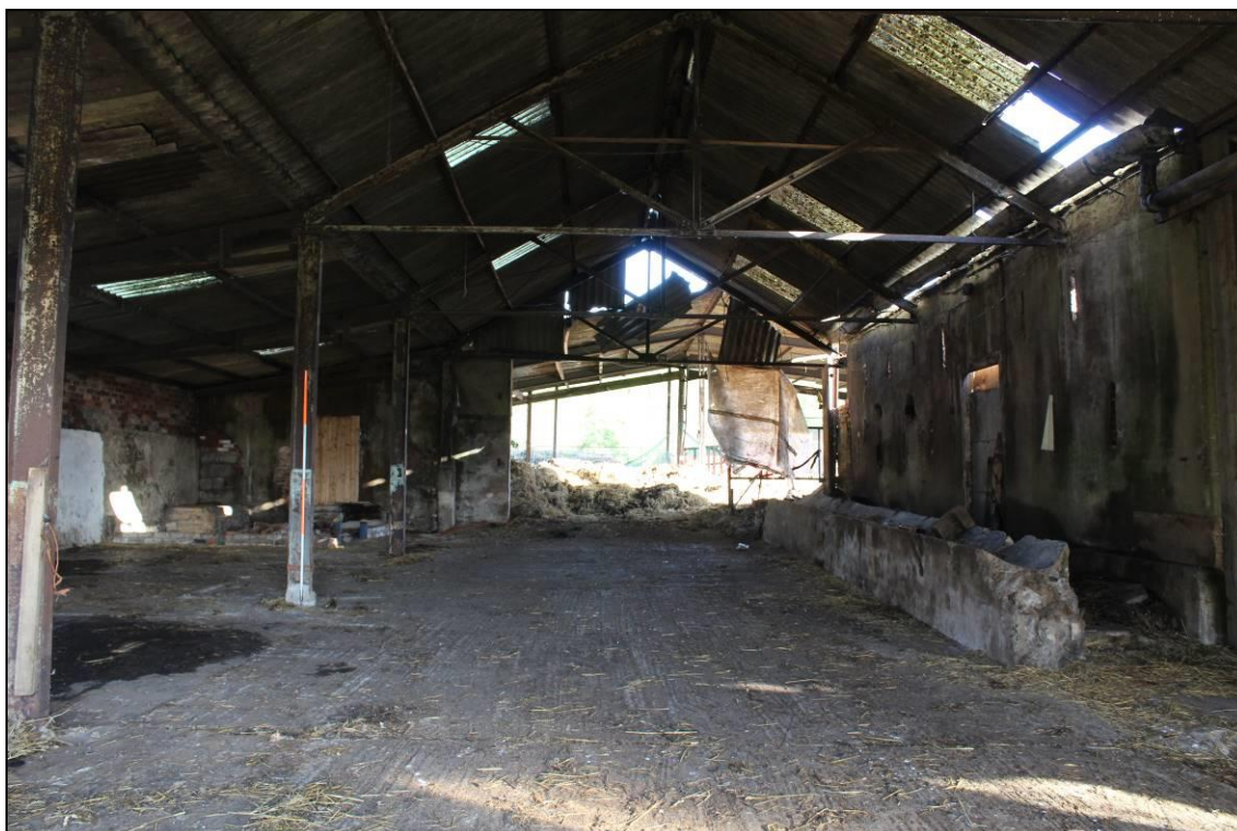
Plate 35: Building B2: interior: view north, 2m scale
