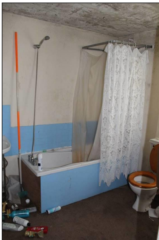
Plate 29: Building A: Room A2.11: view northwest, 2m scale
