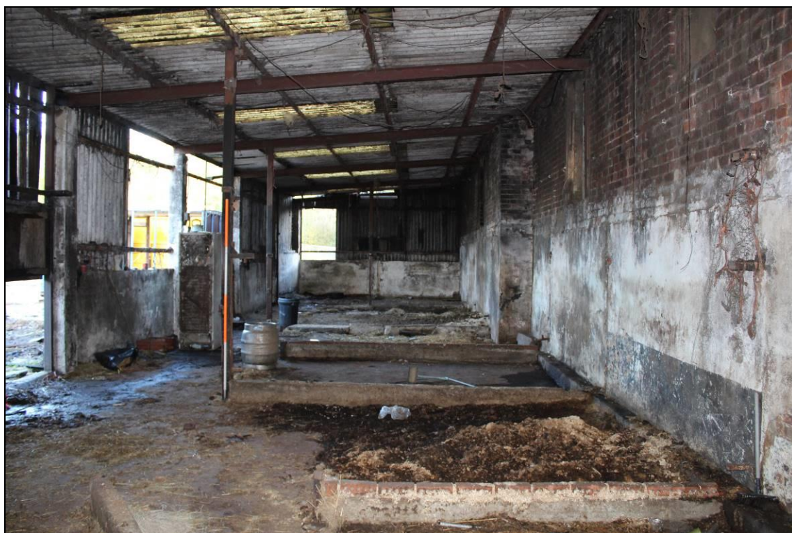
Plate 54: Building C4, south facing elevation (note original sandstone building fabric on lower courses): view northwest, 2m scale
