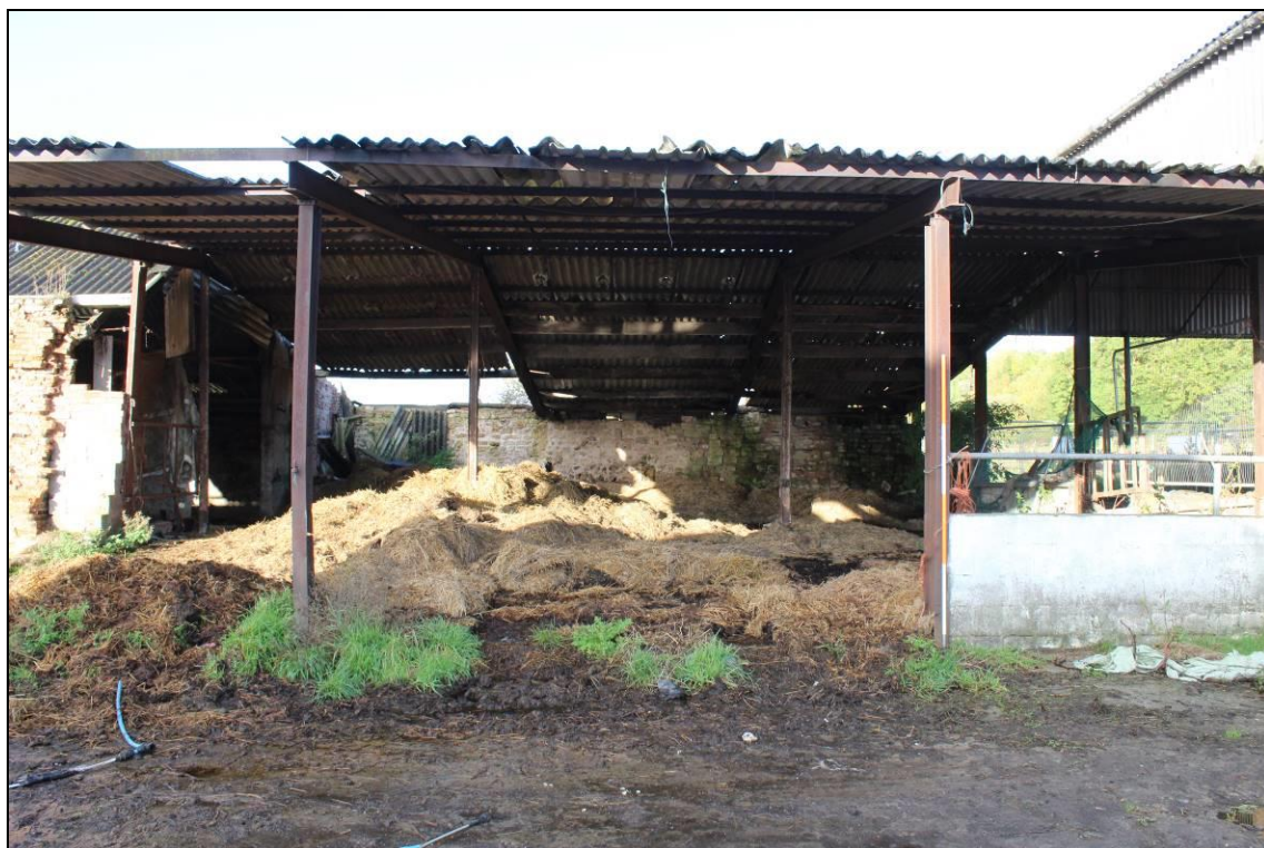
Plate 38: Building B3: Steel portal frame shed: view west 2m scale
