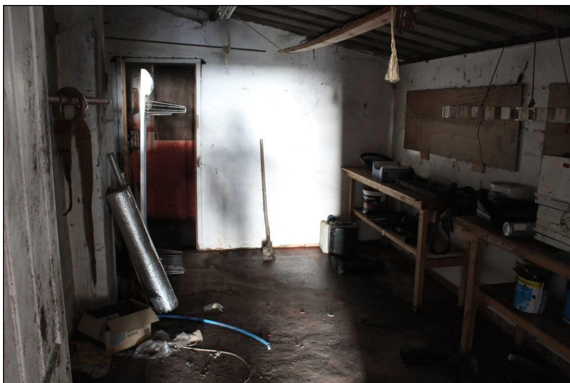
Plate 64: Building E: interior eastern room: view north
