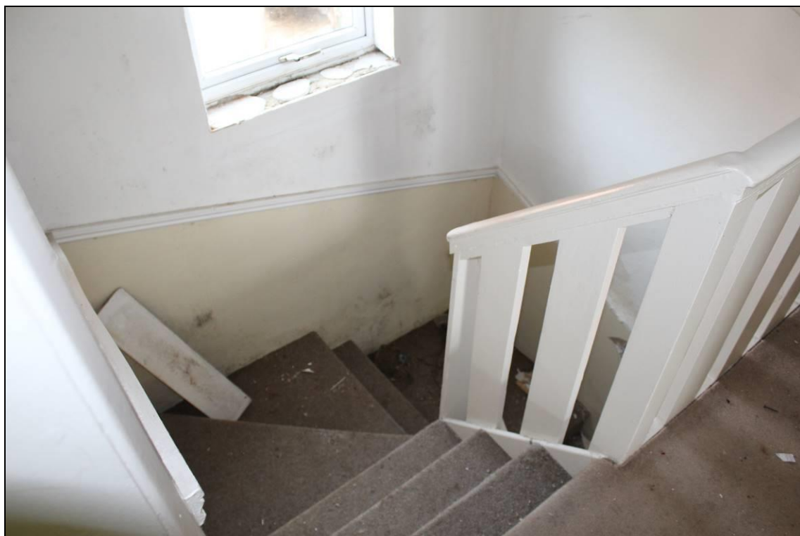
Plate 18: Building A Room A2.1 stairwell: view northeast
