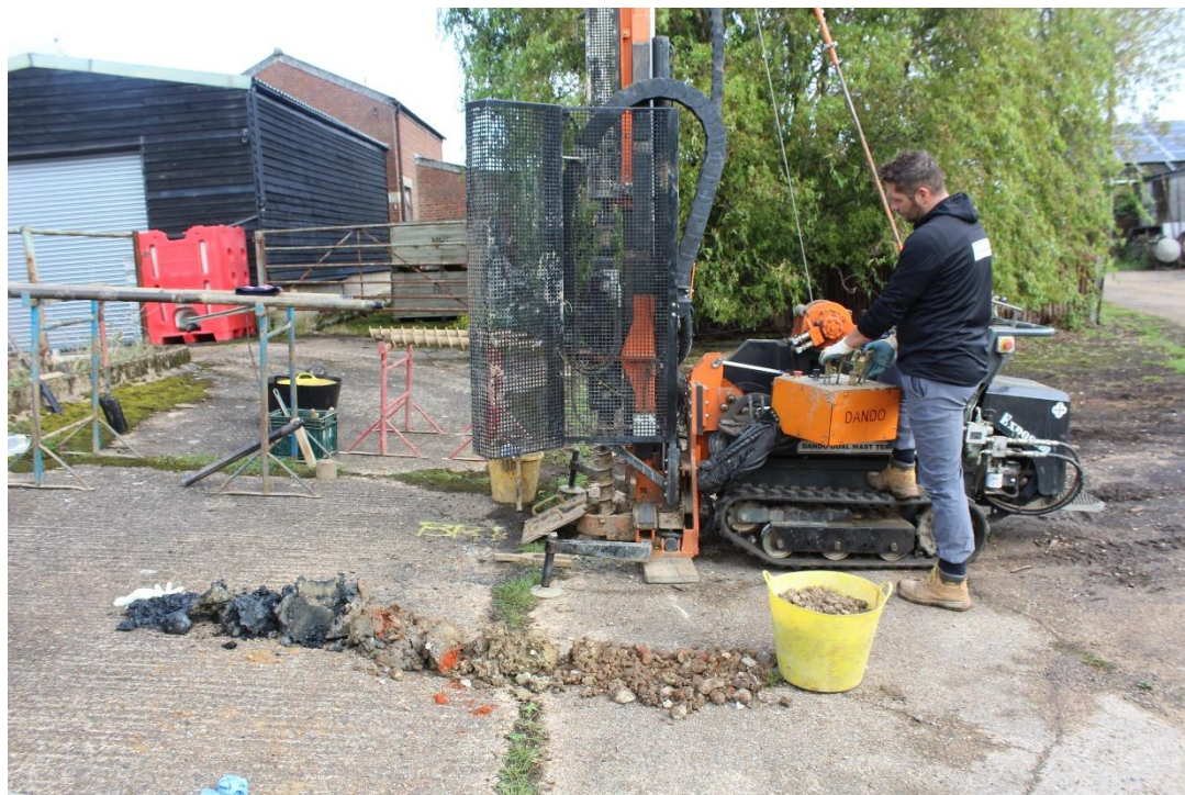
Plate 1: Borehole 1 drilling, looking north
