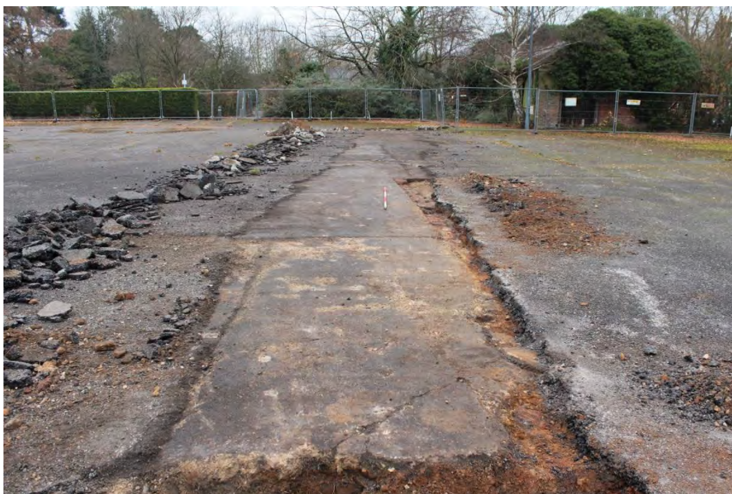
Plate 49: Trench 22 looking east showing concrete surface [33] and wall footing [34], 2m scale
