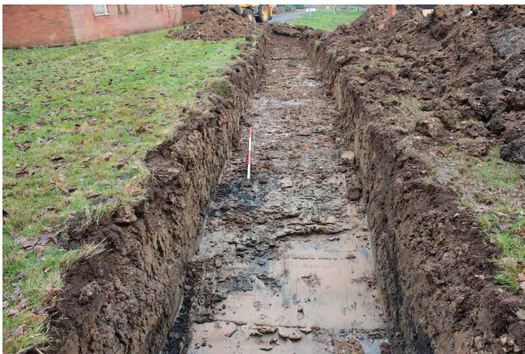
Plate 9: Trench 5 looking west showing made ground [126], 2m scale
