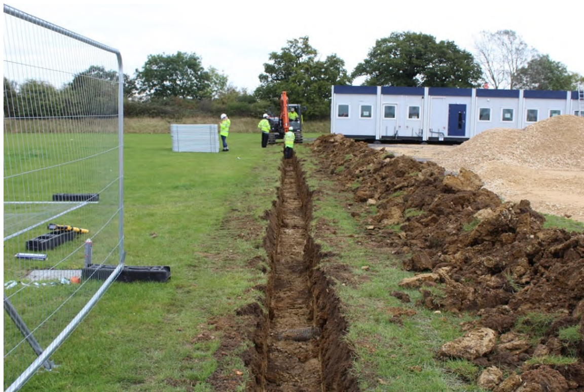
Plate 3: Pavement and utility trench facing east
