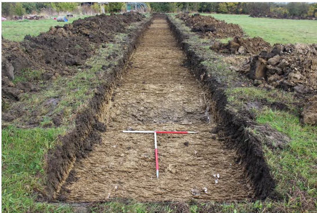
Plate 1: Trench 1, view NE. Road [131] (before excavation) visible in the middle of the trench.
