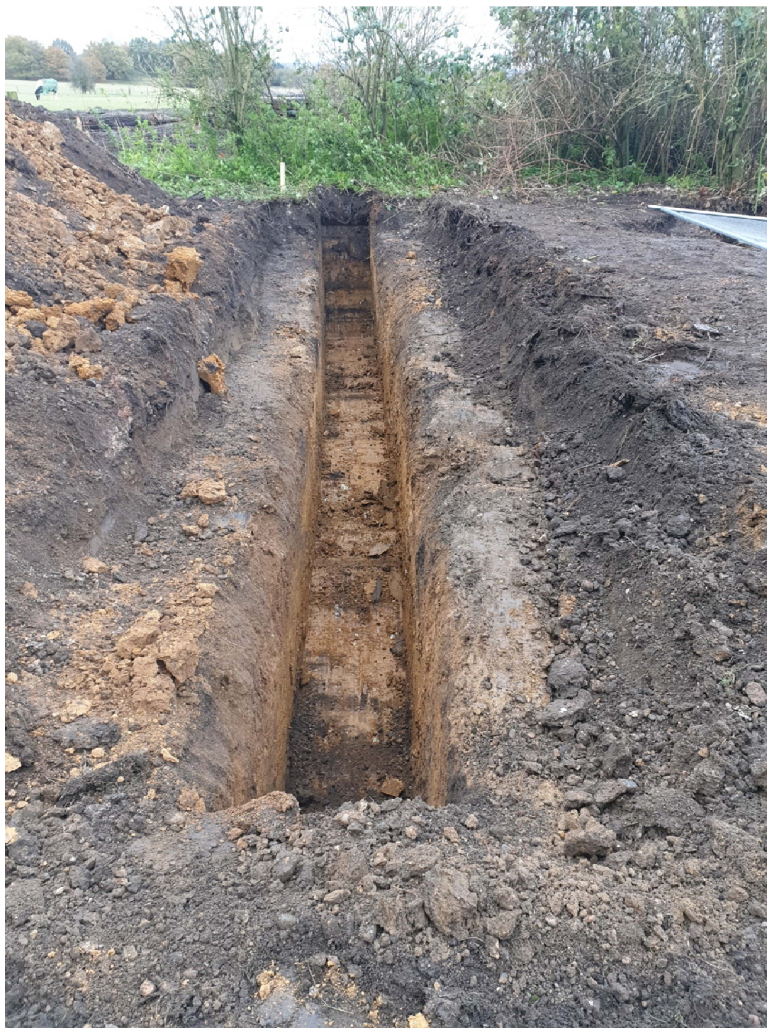
Plate 3 East footing facing south-east
