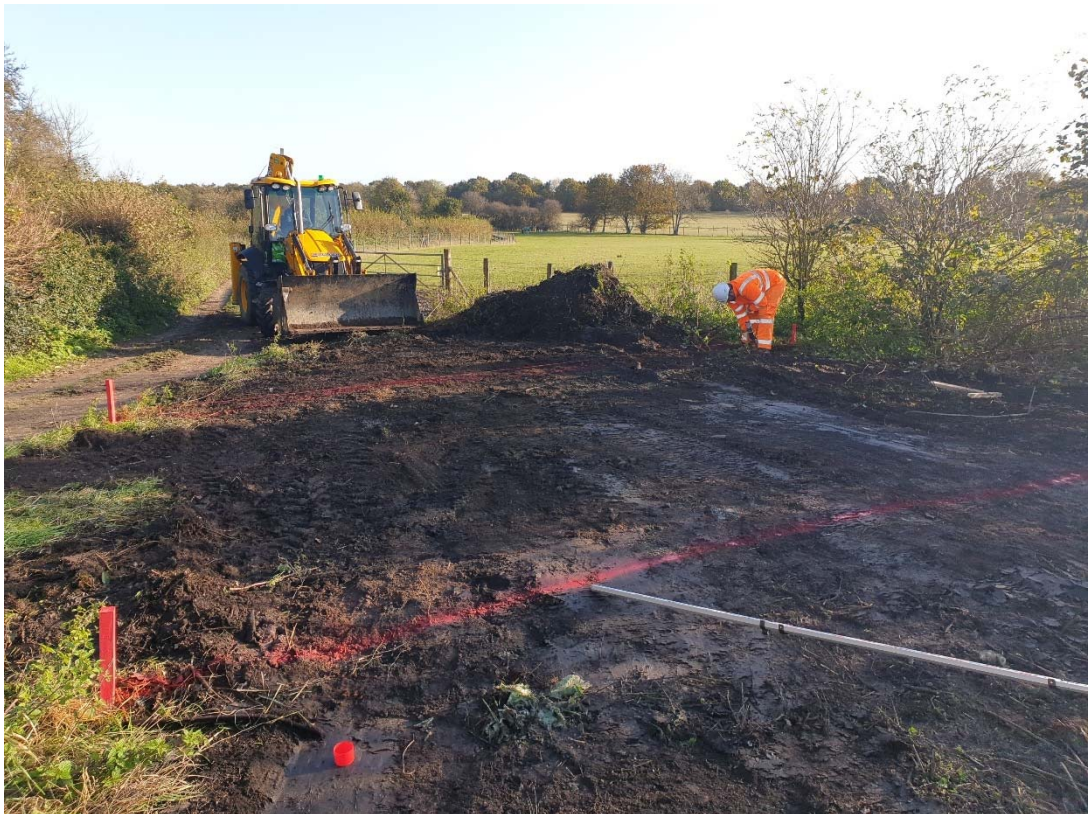
Plate 2 Working shot facing east
