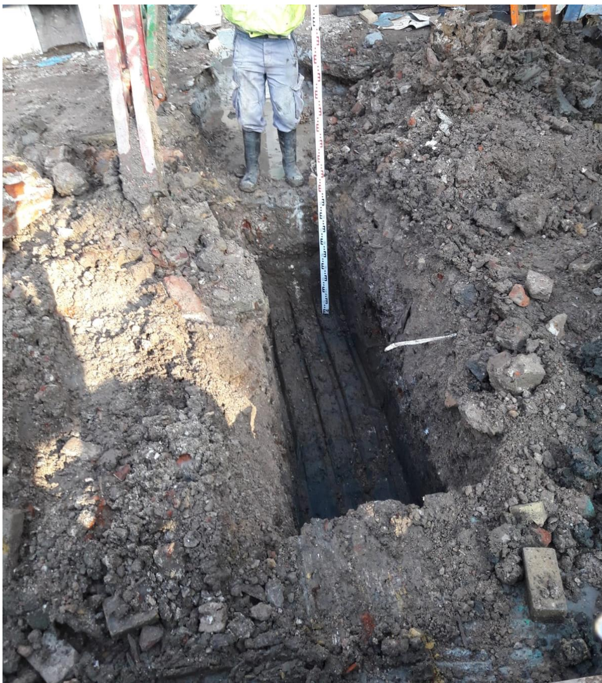
Plate 1: Photograph provided by DB Construction, foundation trench, looking north.
