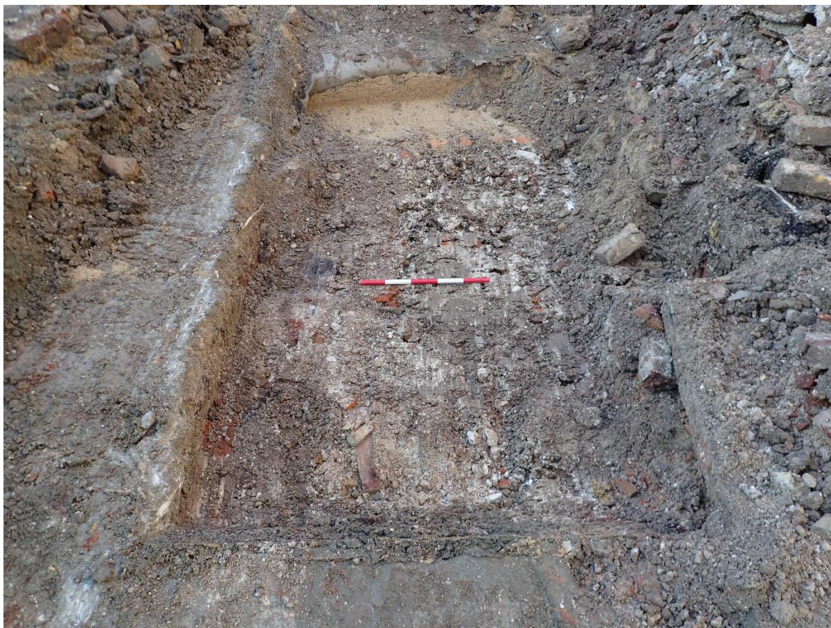
Plate 3: Bay 2, looking west, modern plastic ducting laid in sand in the background with demolished wall [3] on the left in the foreground, 0.5m scale
