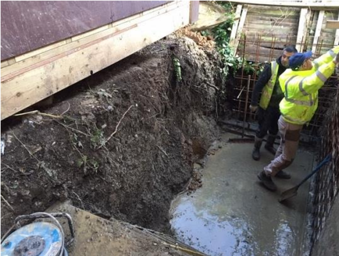
Plate 1: View to east of underpinning at eastern boundary
