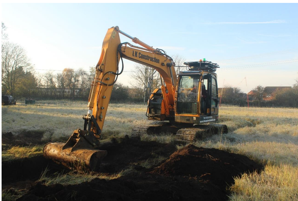
Plate 2: Working shot; view south-west
