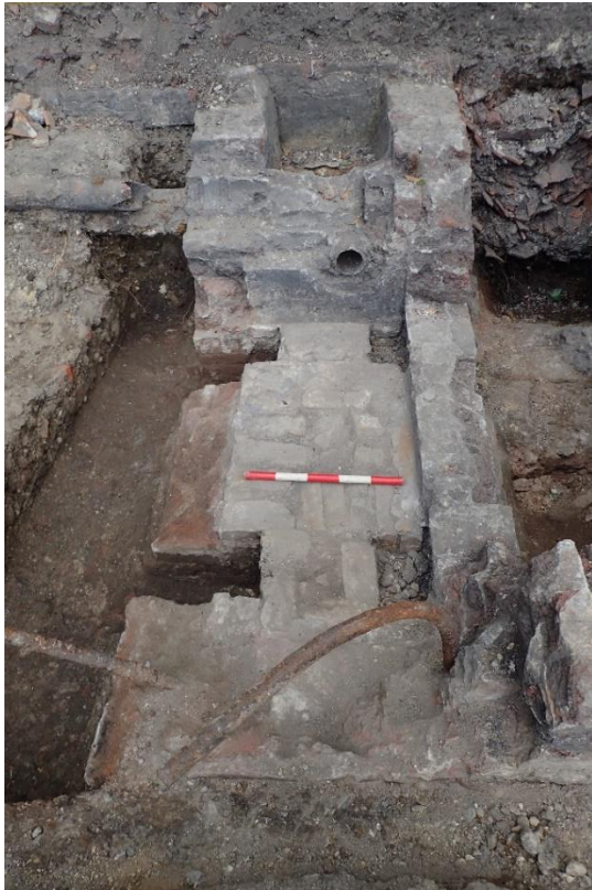
Plate 11: Brick tank [118] with pipes leading into a missing structure supported on brick base [119] to the south-east. Note the pipes leading out of tank [118] to the south-west and under floor [101]. Looking north-west (0.5m scale)
