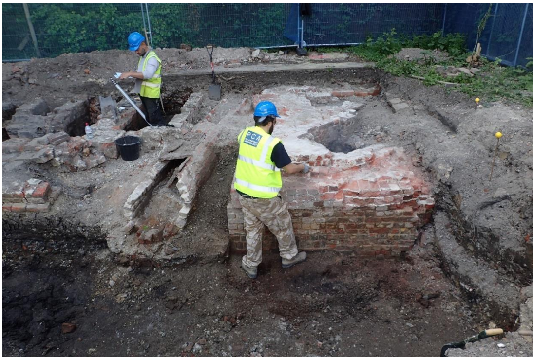
Plate 2: Phase 2 brick base foundation [140] and [126] to the dye furnaces, showing the slightly different alignment of the two parts of this structure, looking north-west.
