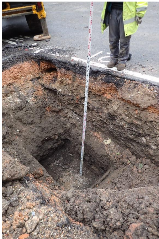
Plate 2: Trench 1 sondage, north facing view
