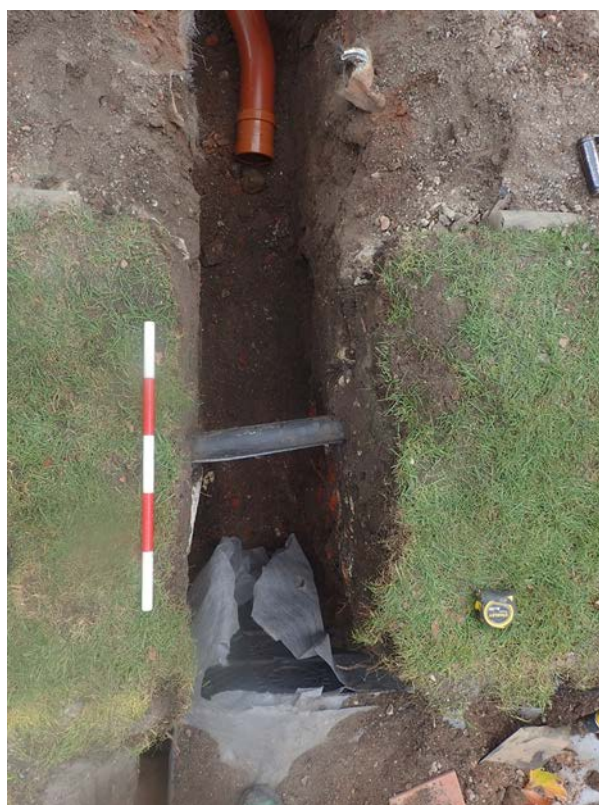
Plate 6: TP1, Connecting the drainage , looking North
