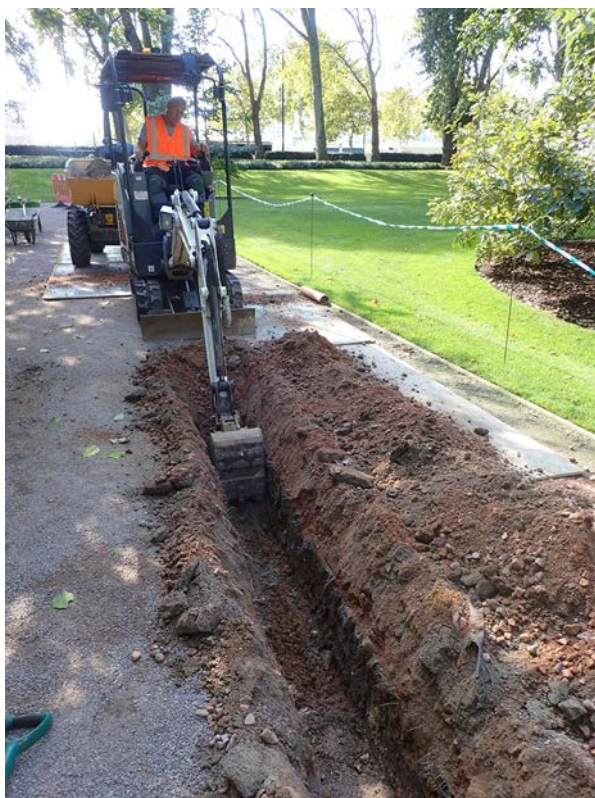
Plate 5: Excavation of Western Pipe Trench, looking South
