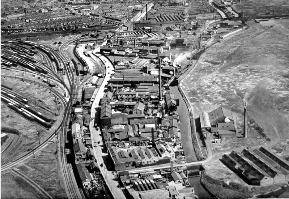
Plate 1 Oblique aerial photograph of Carpenter's Road, looking south-east, c 1930
