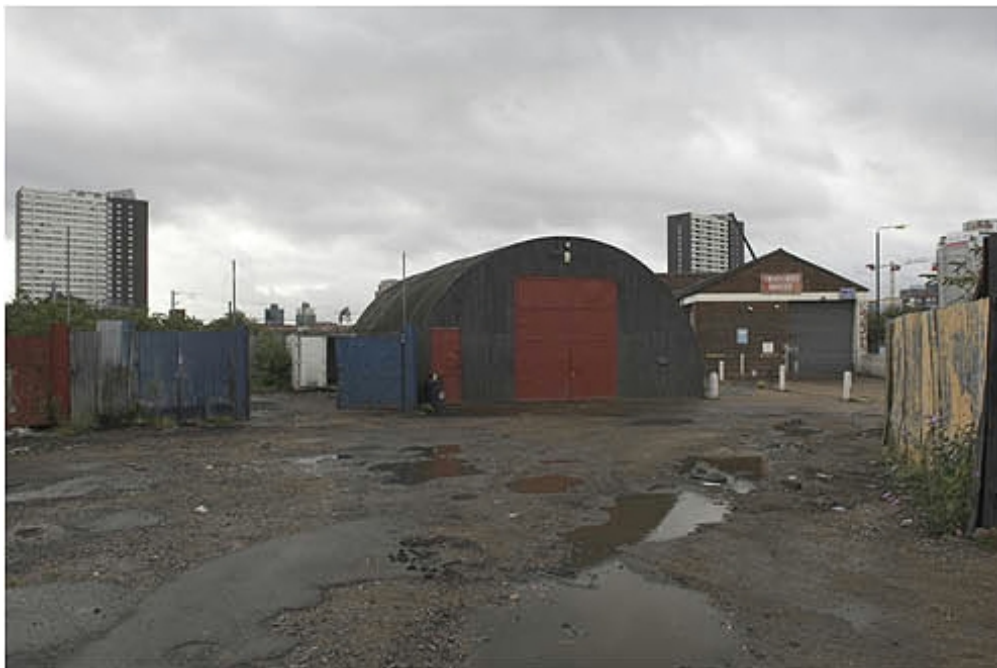
Plate 8 View of Building 3, looking north – north-west
