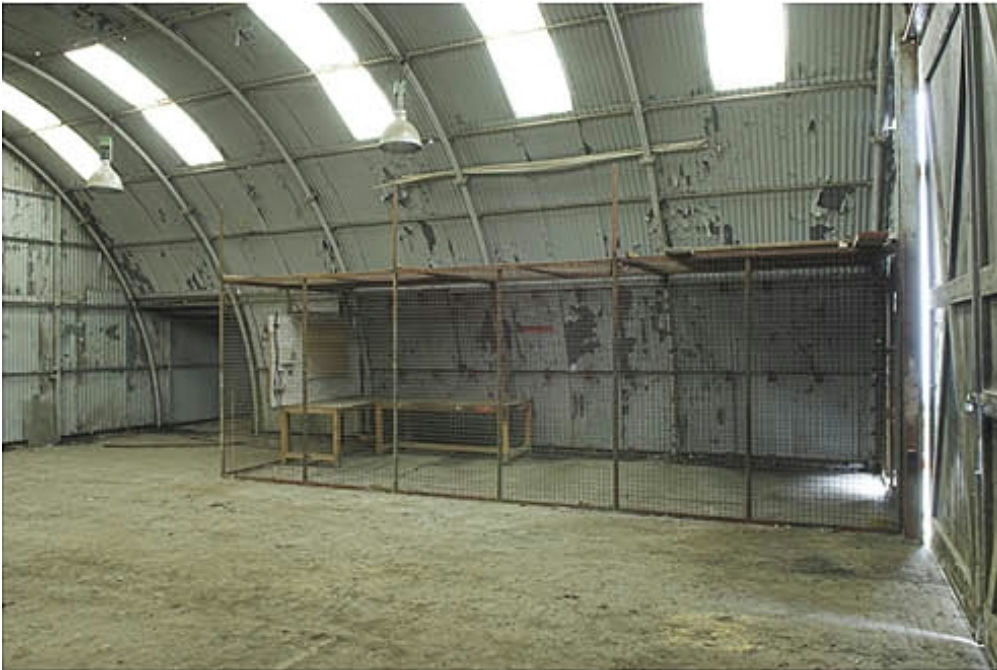
Plate 6 View of Building 2, showing covered way, looking north-east
