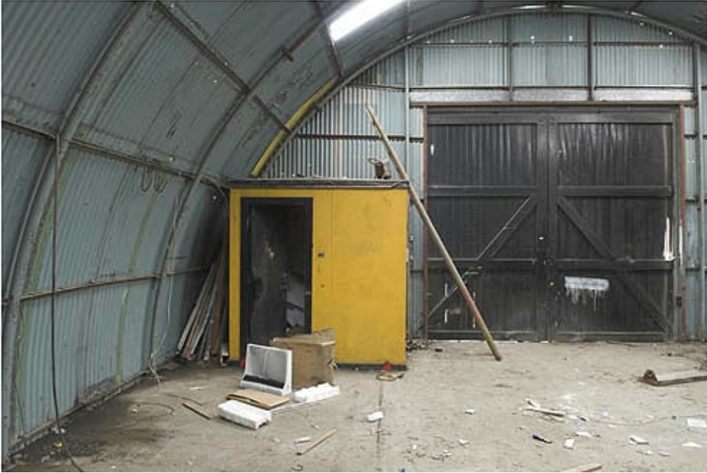
Plate 4 View of Building 1, gable end and timber unit, looking north-west
