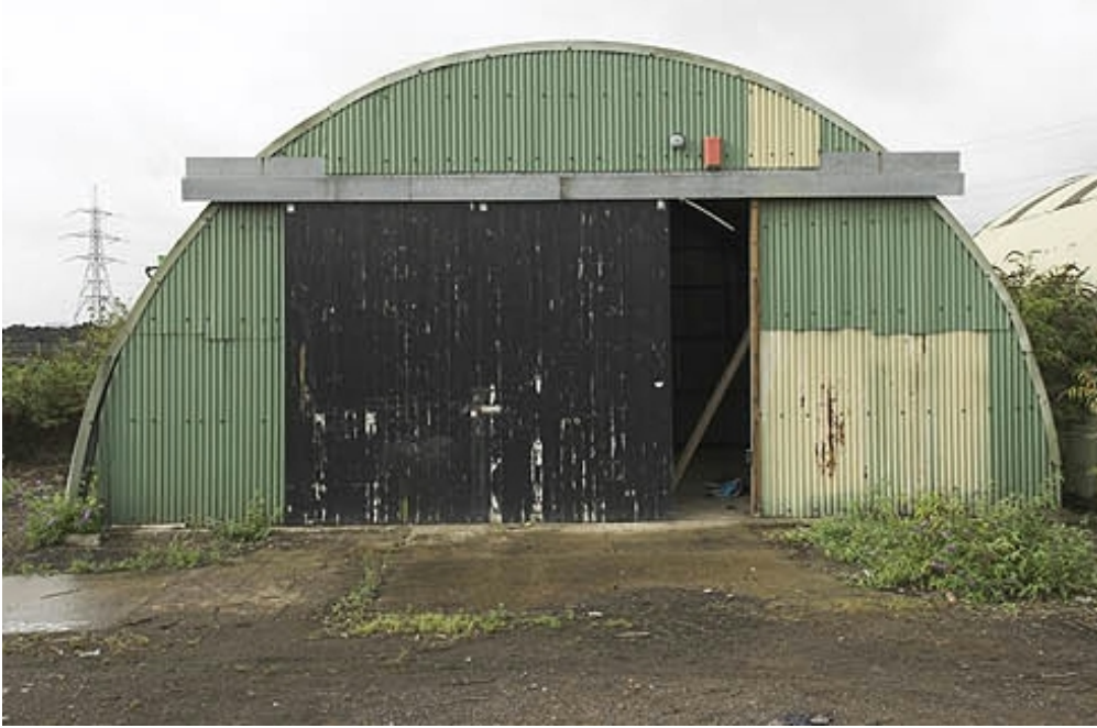
Plate 2 View of Building 1, gable end, looking north
