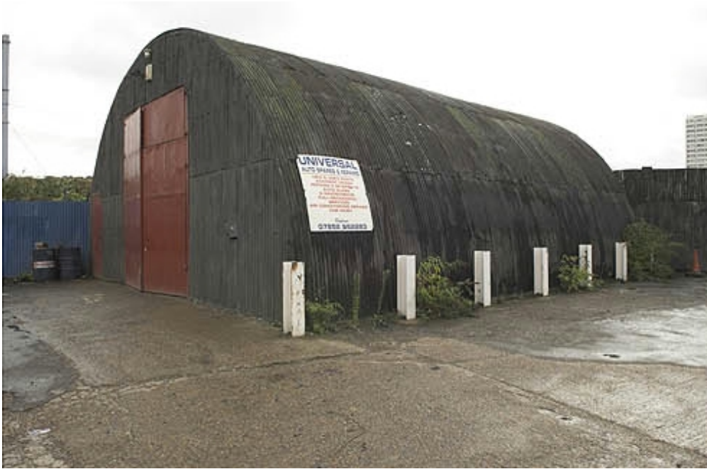
Plate 7 View of Building 3, looking west
