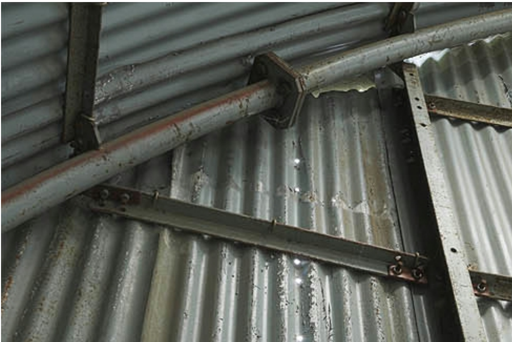
Plate 3 View of Building 1, detail of main rib, angle purlins and hooks
