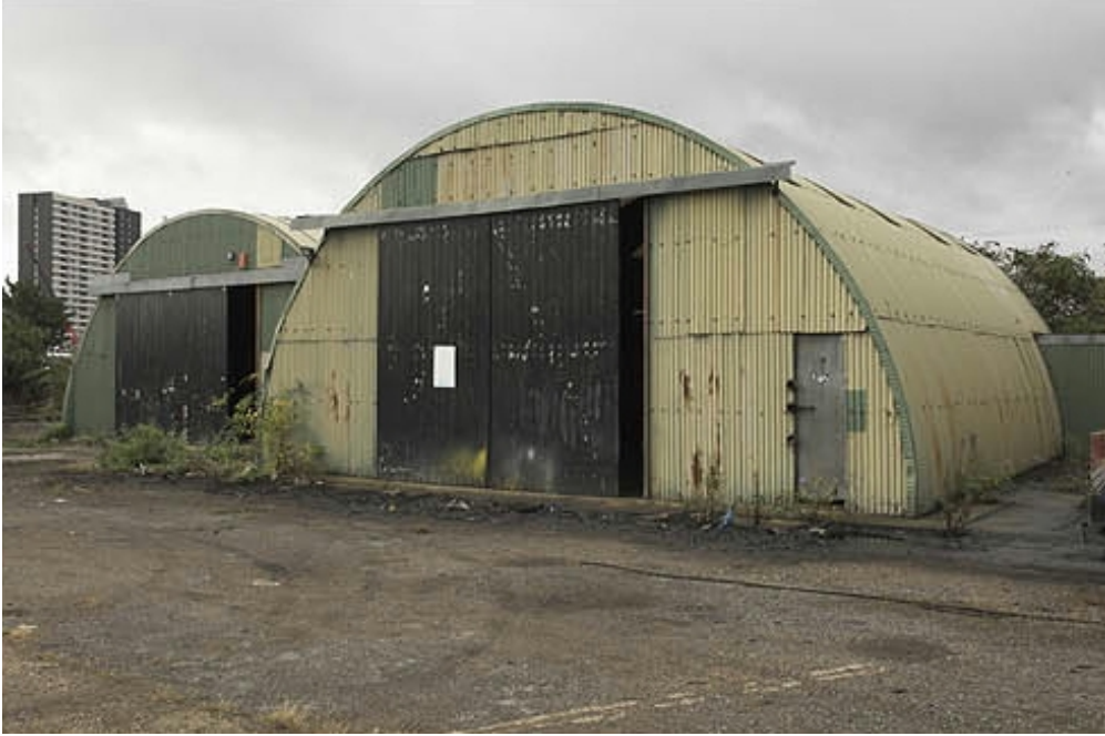
Plate 5 View of Building 1 and 2, gable ends, looking north - north-west
