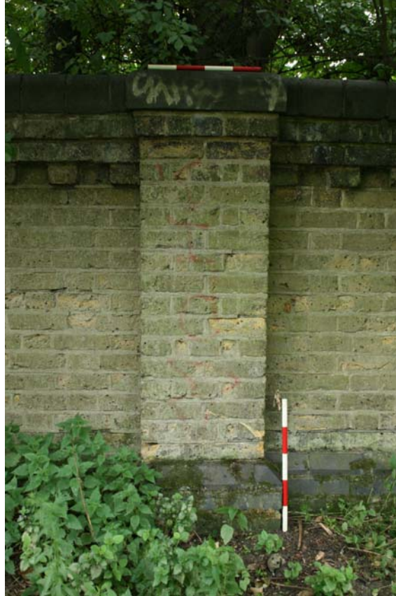
Plate 16 Typical buttress showing brick detailing, west side of wall. Scale 5x100mm
