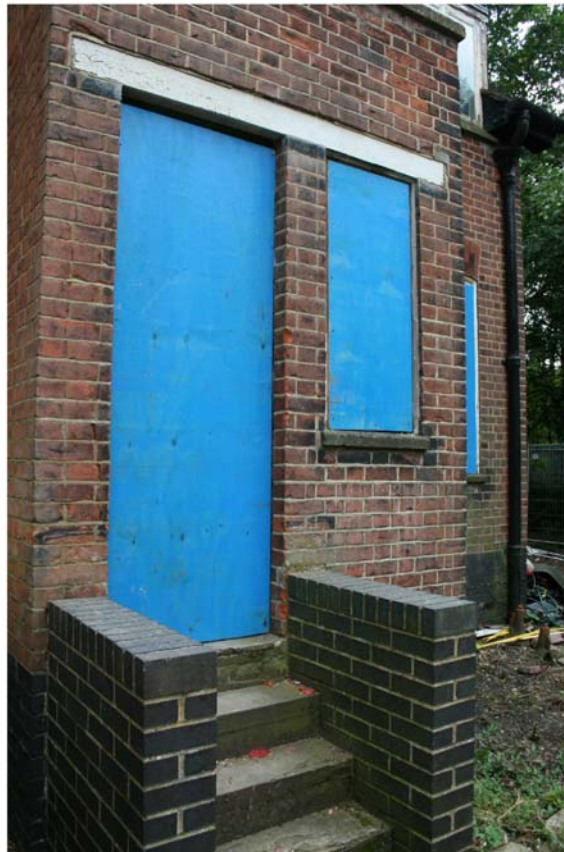
Plate 2 Front door of cottage, western elevation
