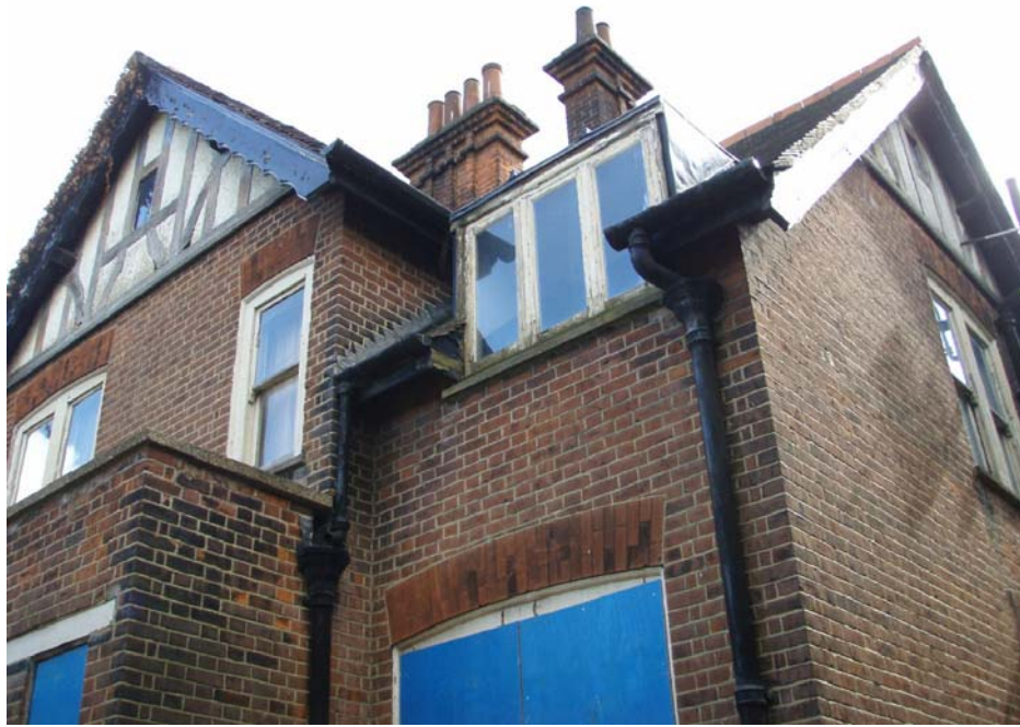
Plate 1 View of cottage from south-west, showing roof form and half-timbered gables
