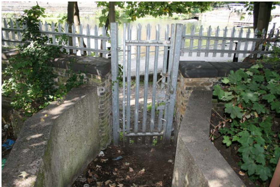
Plate 19 Midpoint opening in wall
