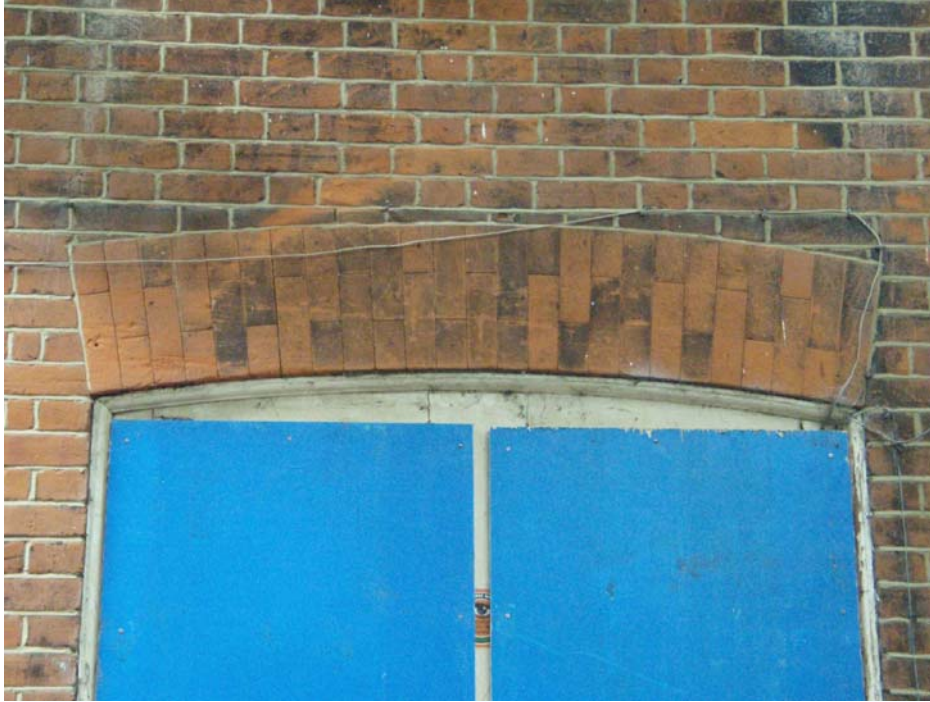
Plate 4 Typical brick-arched window head
