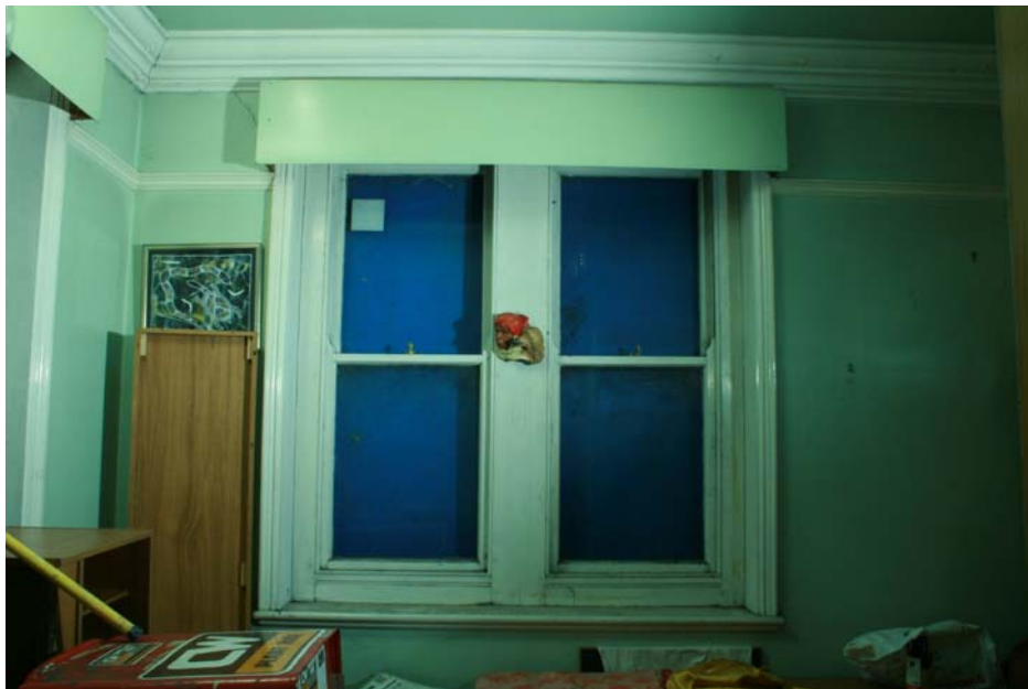
Plate 12 Window in room at north-west of cottage, looking north
