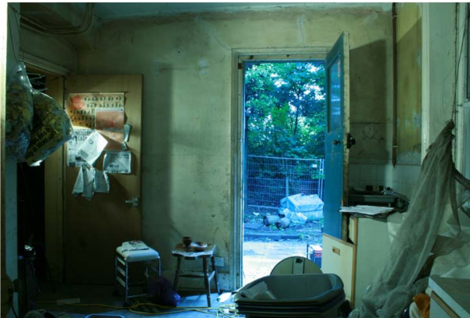
Plate 6 Kitchen, looking east
