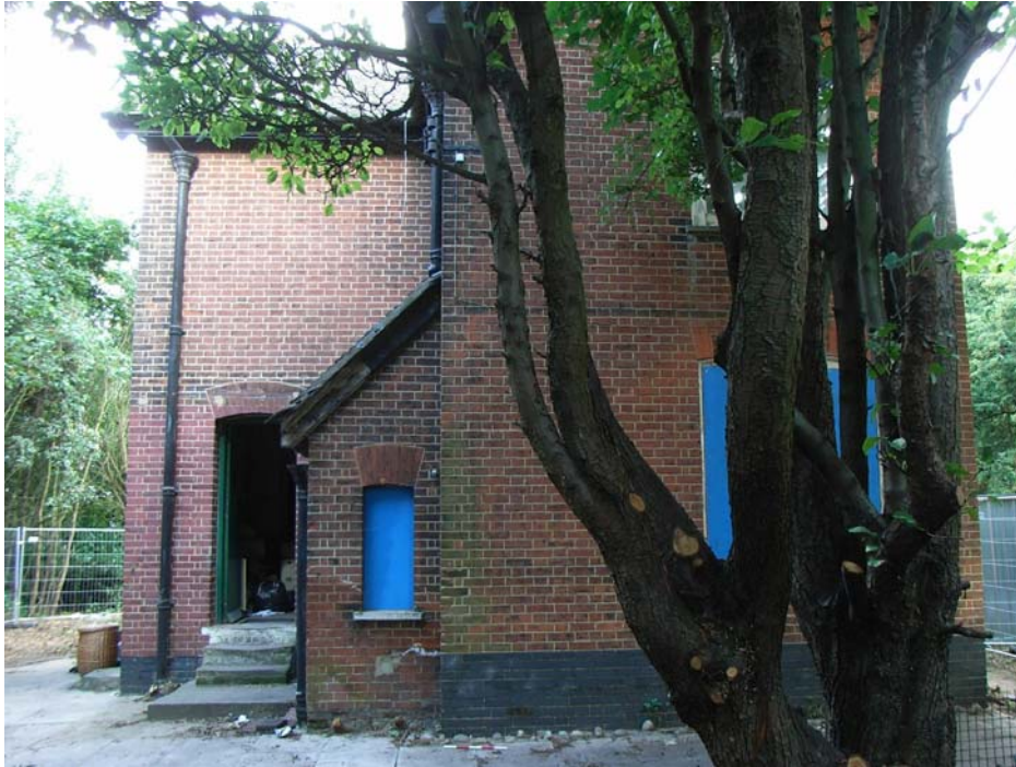
Plate 5 East elevation of cottage
