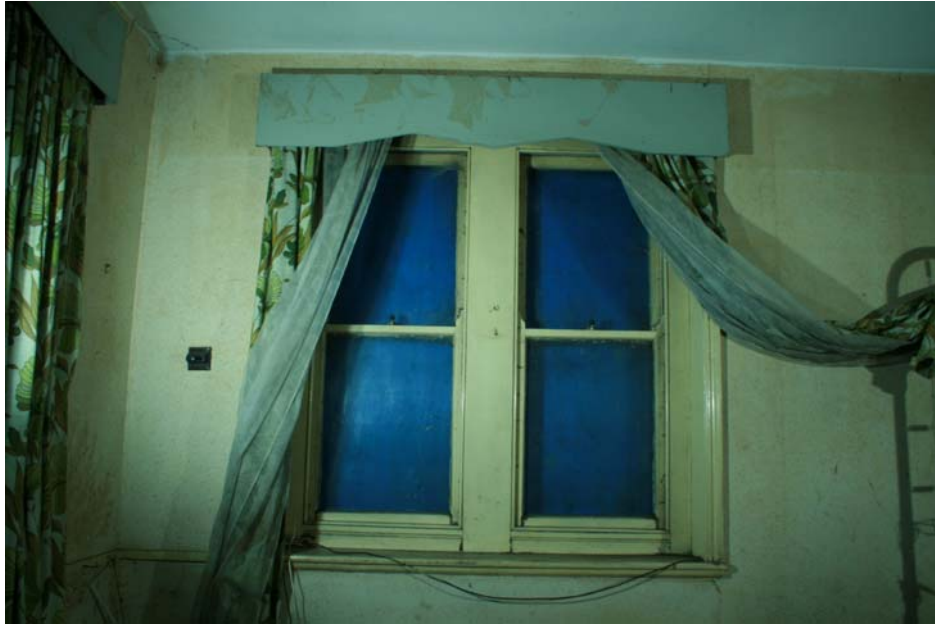
Plate 10 Window in east wall of north-east room, looking east
