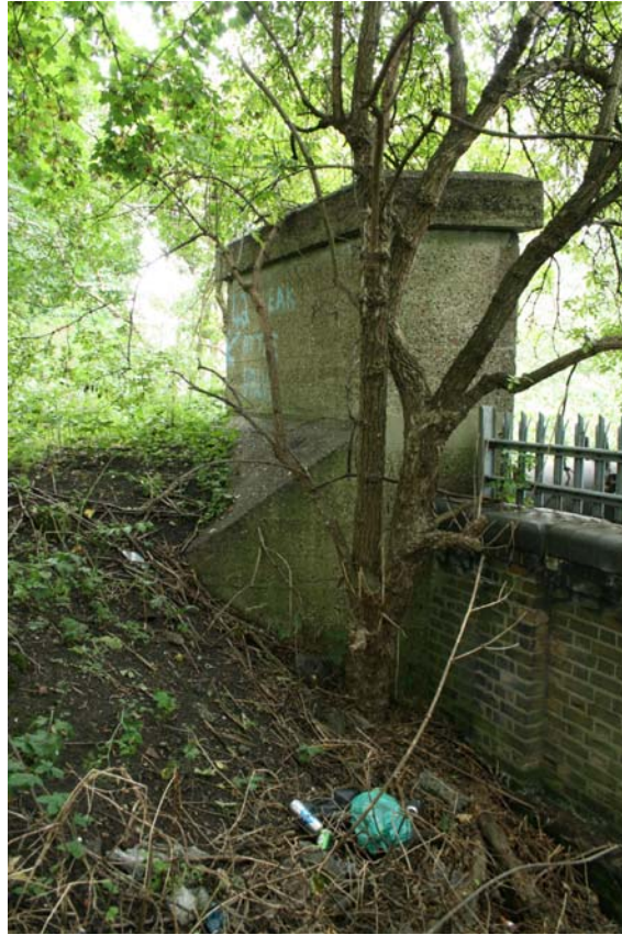
Plate 20 Concrete structure containing pipes extending over River Lea
