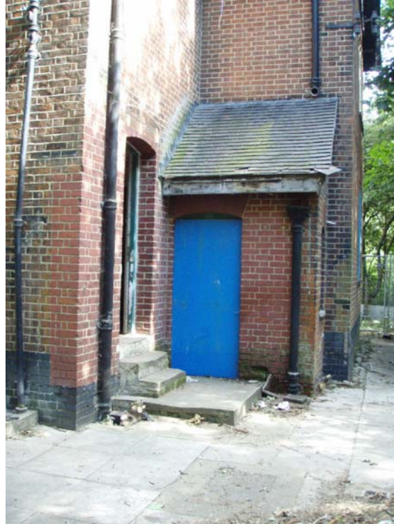
Plate 3 Back door and outhouse, eastern elevation
