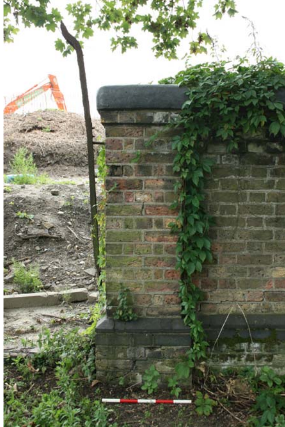
Plate 21 Northernmost opening in wall, showing truncated metal gatepost. Scale 5x100mm
