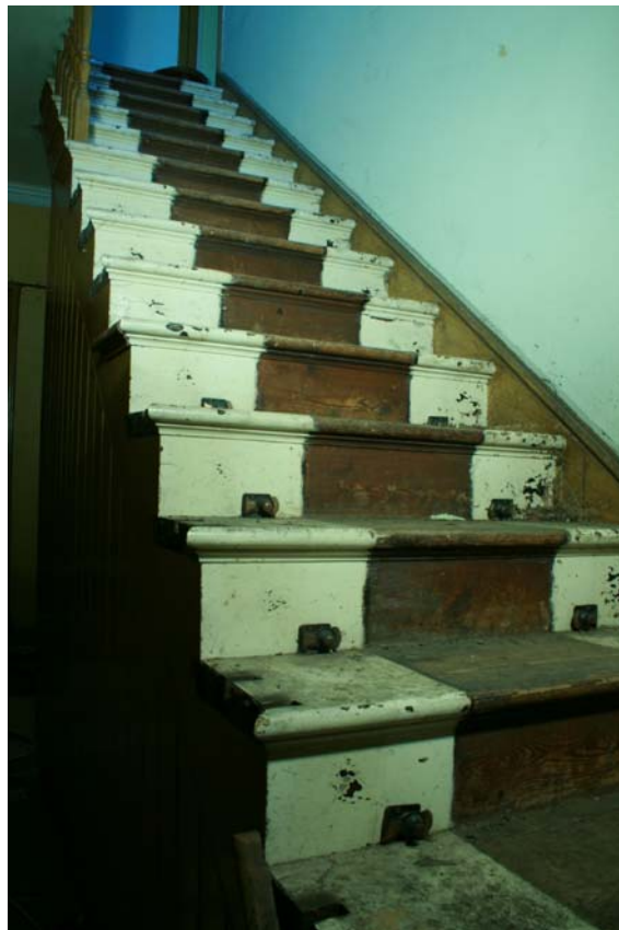
Plate 11 Staircase, looking south-east
