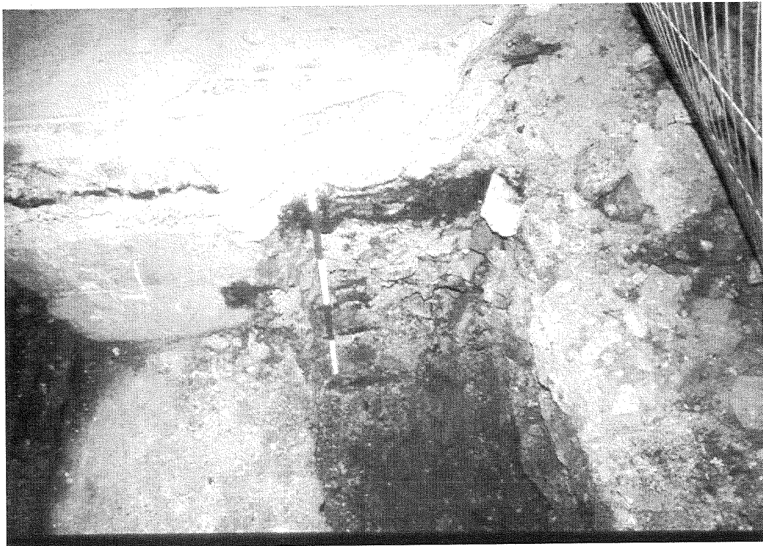
Plate 15. View of foundations in Trial Pit 07
