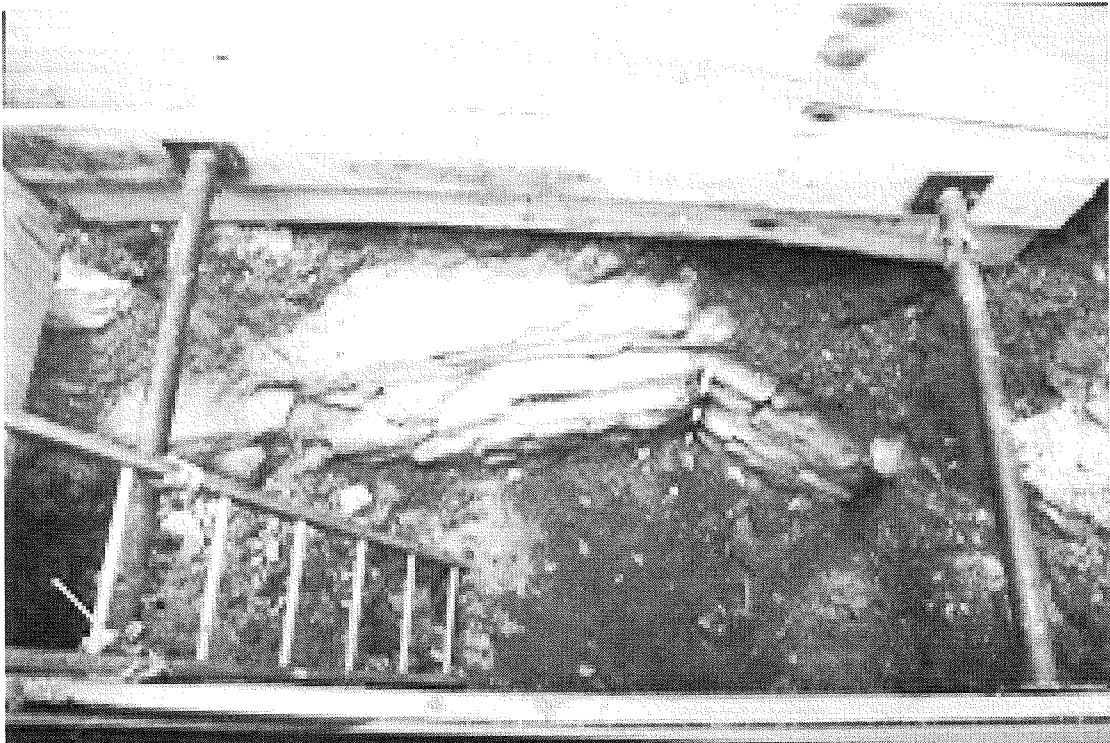
Plate 14. View of wall foundation of no. 9 Bath Street in Trial Pit 03.
