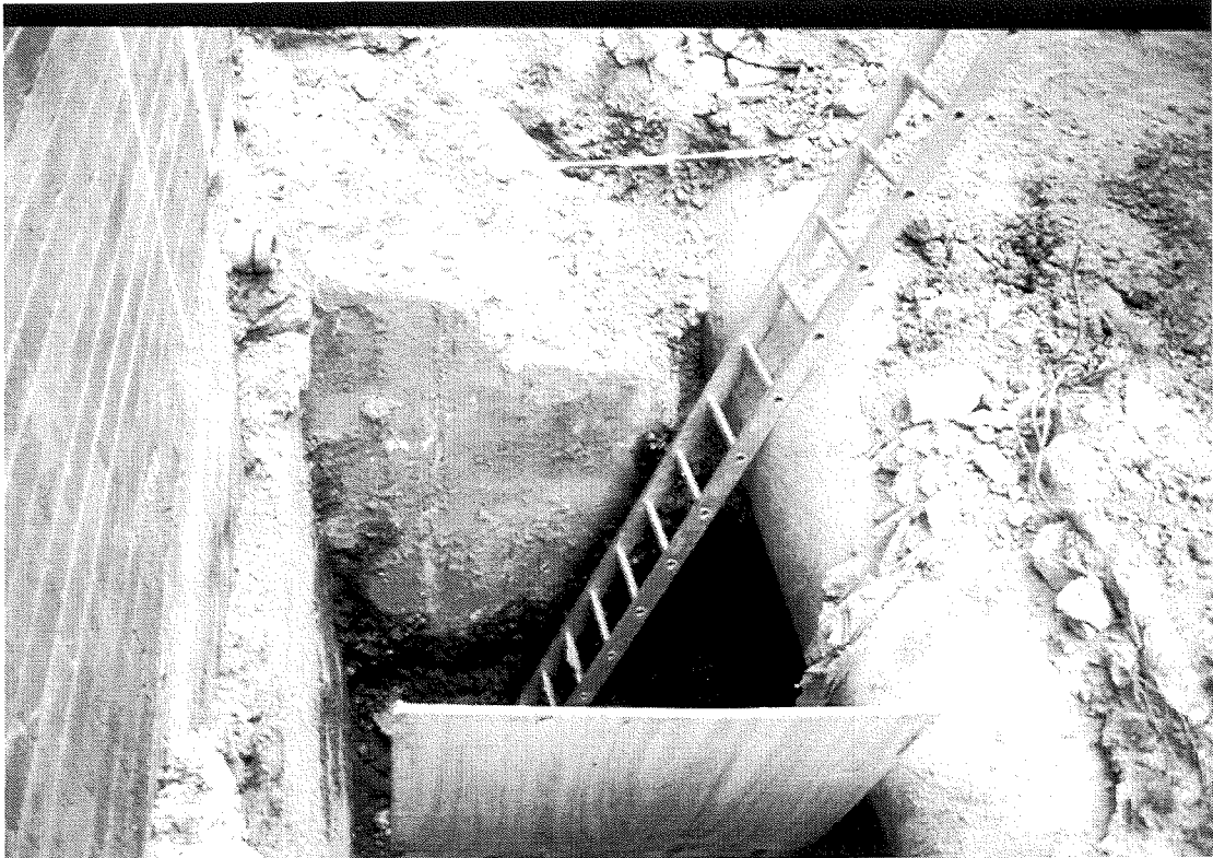
Plate 20. View of gas main in Trial Pit 15.
