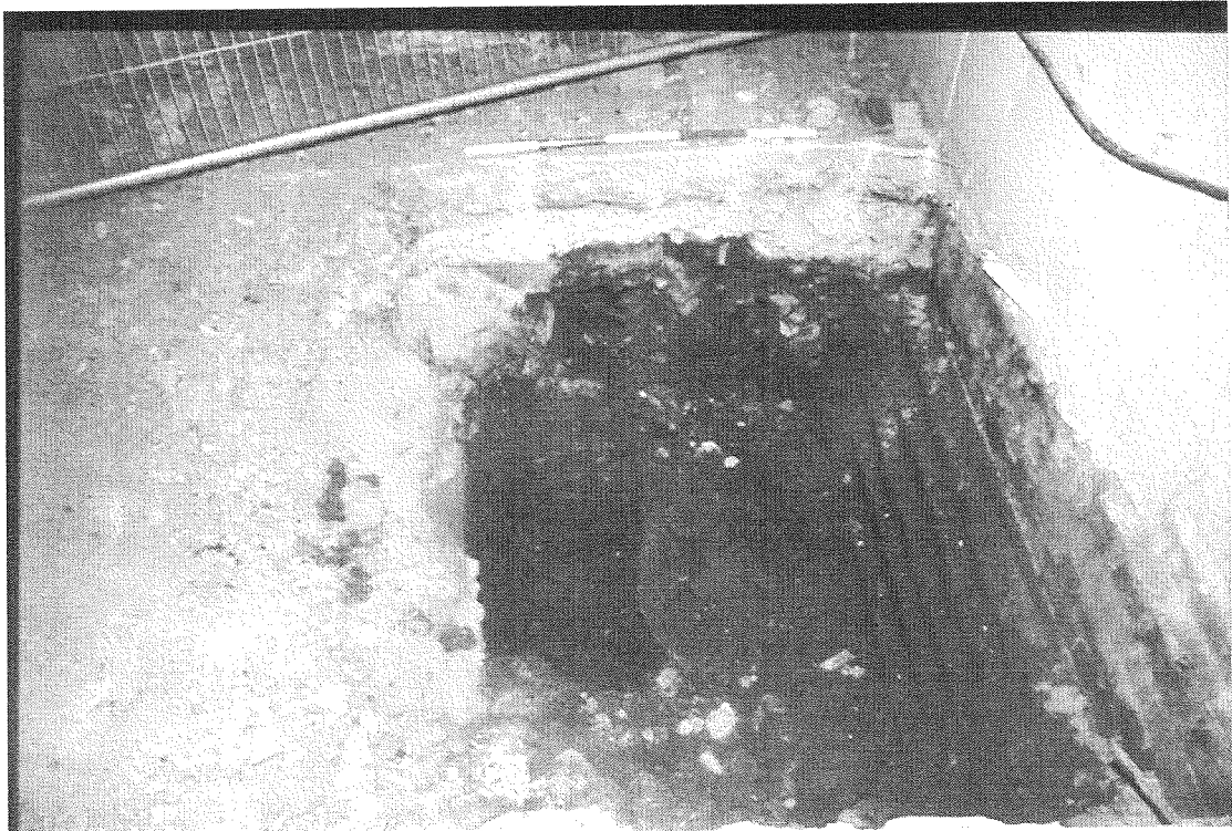
Plate 16. View of Old Fermentation Building Foundations in Trial Pit 08
