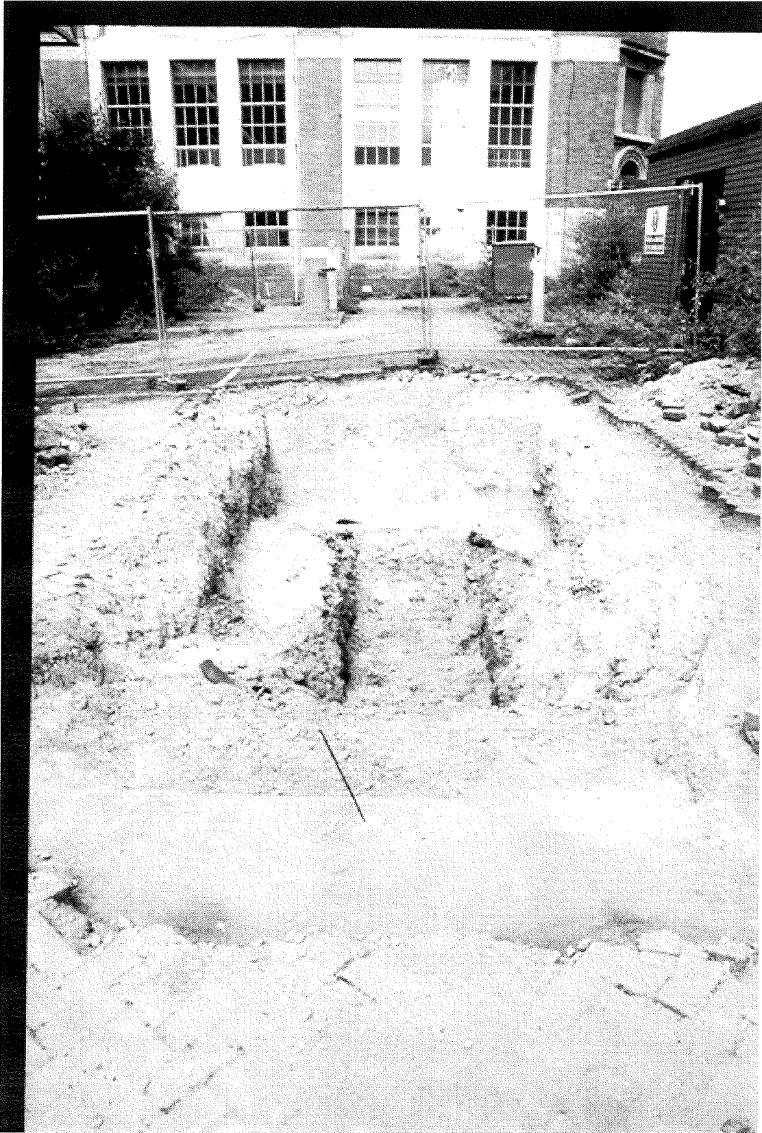
Plate 3. View of Trench 22 from the south-west.
