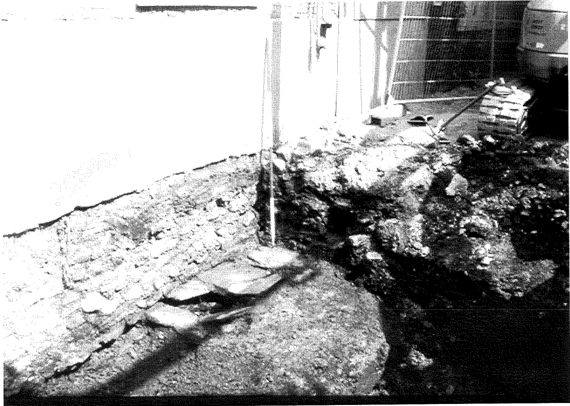
Plate 17. View of Old Compressor Building foundations in Trial Pit 09/10.
