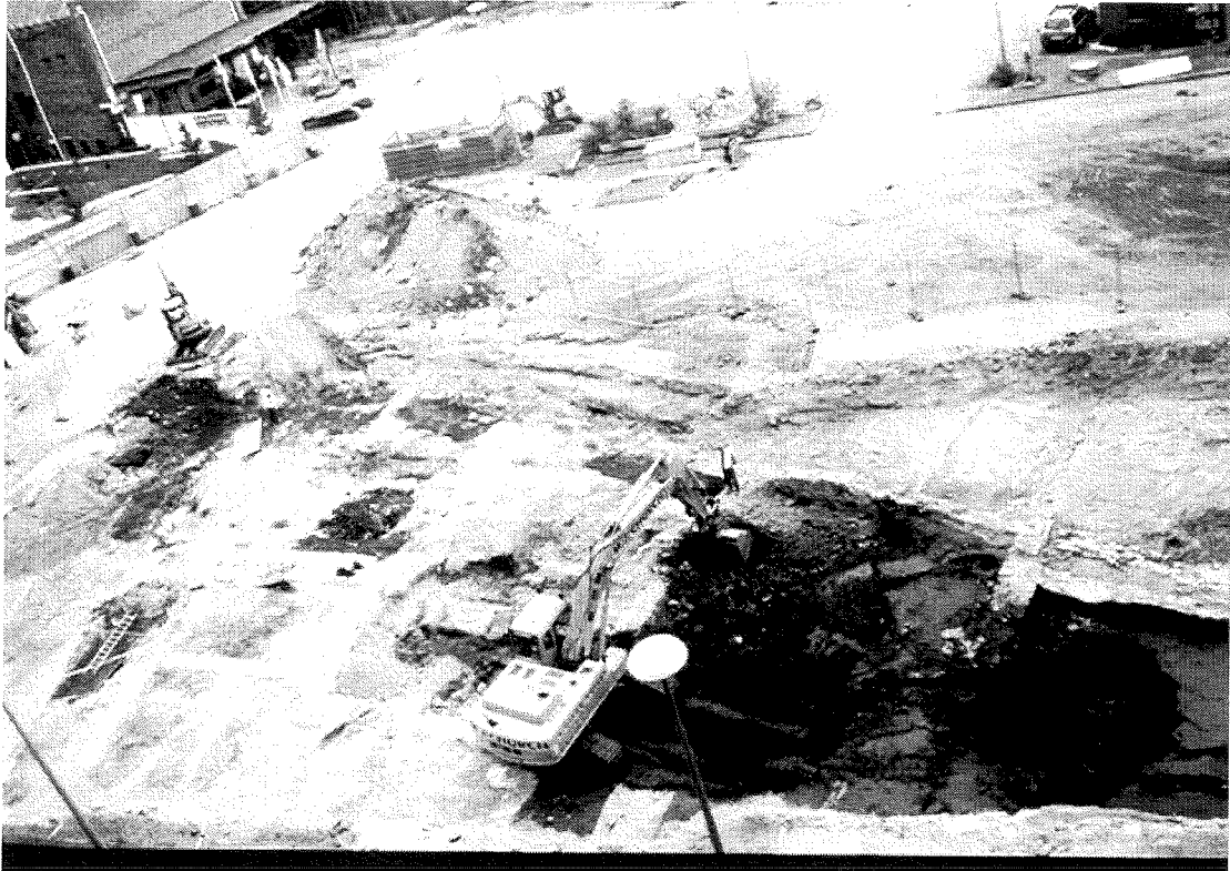
Plate 8. View of northern part of Trench 26.
