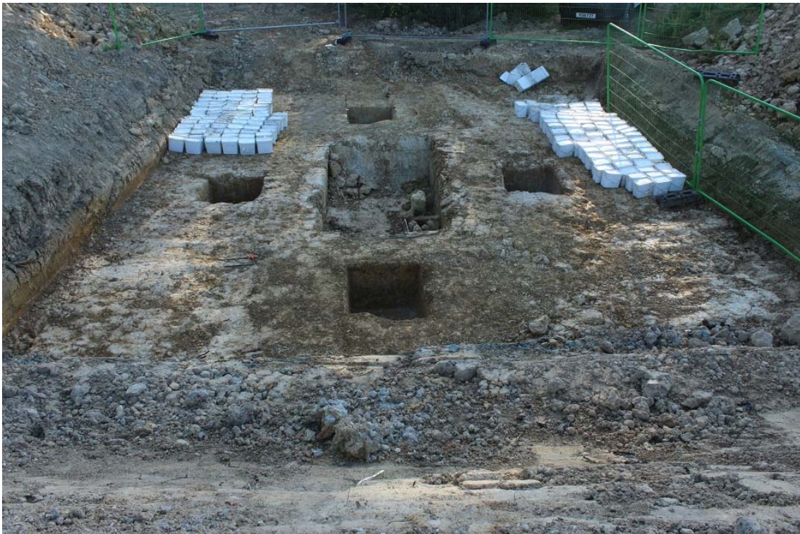
Plate 10. Test pits in area 2, view east
