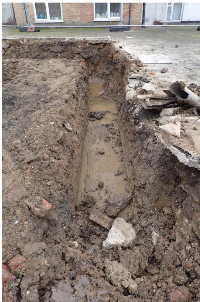
Figure 1: Clay [2] in base of trench
