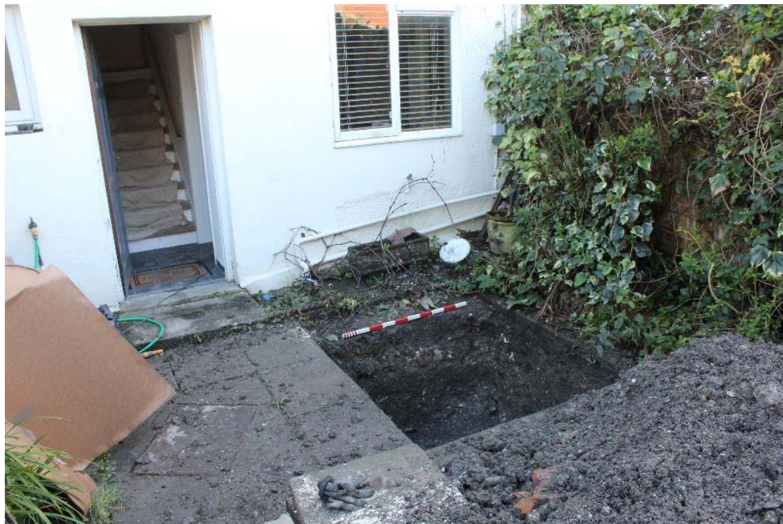
Plate 1. Overview of test pit 1, looking south east. Scale 1m.
