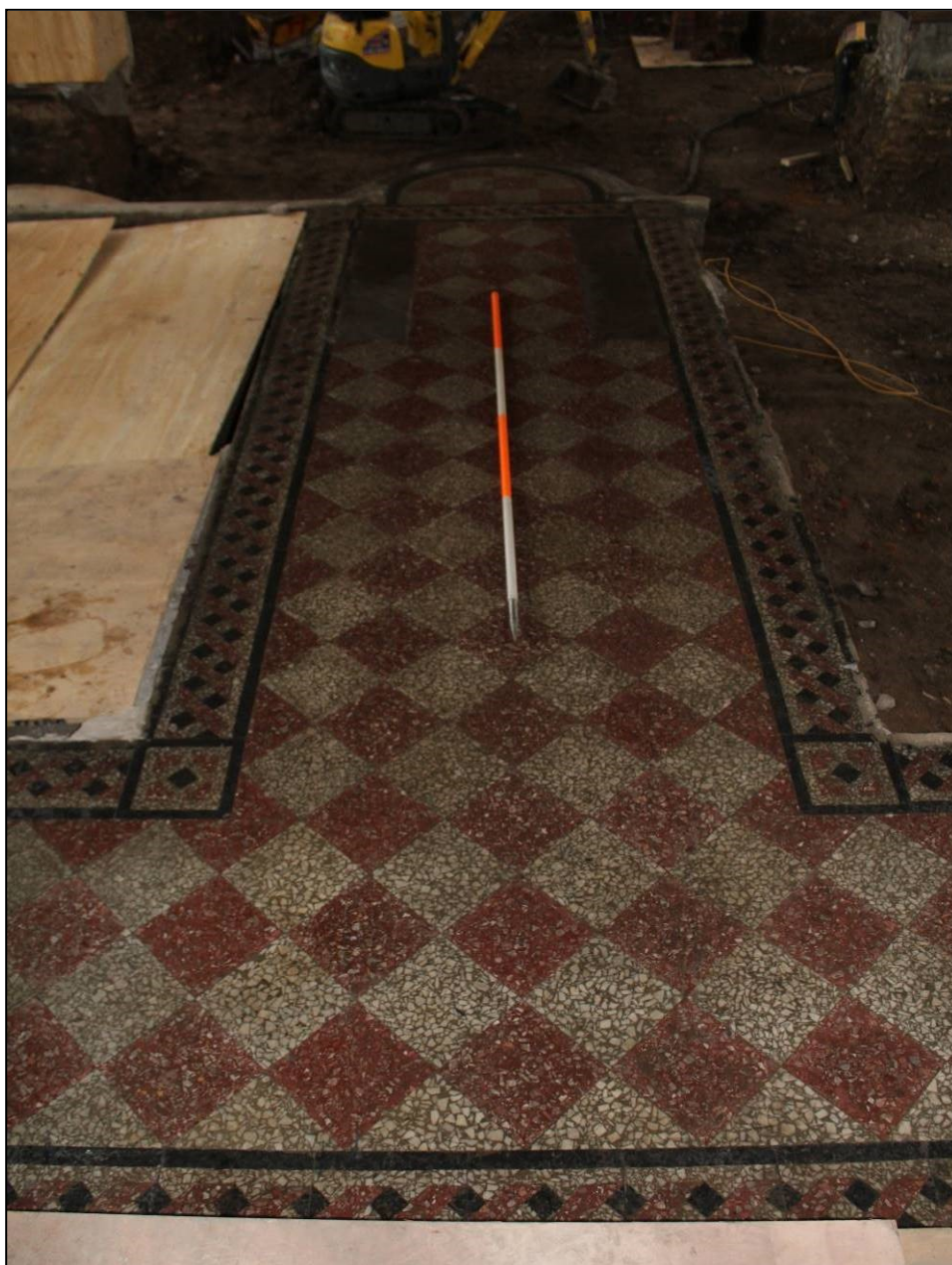
Plate 23: Tiled floor surface [200] within dais/chancel: view southwest, scale: 2m
