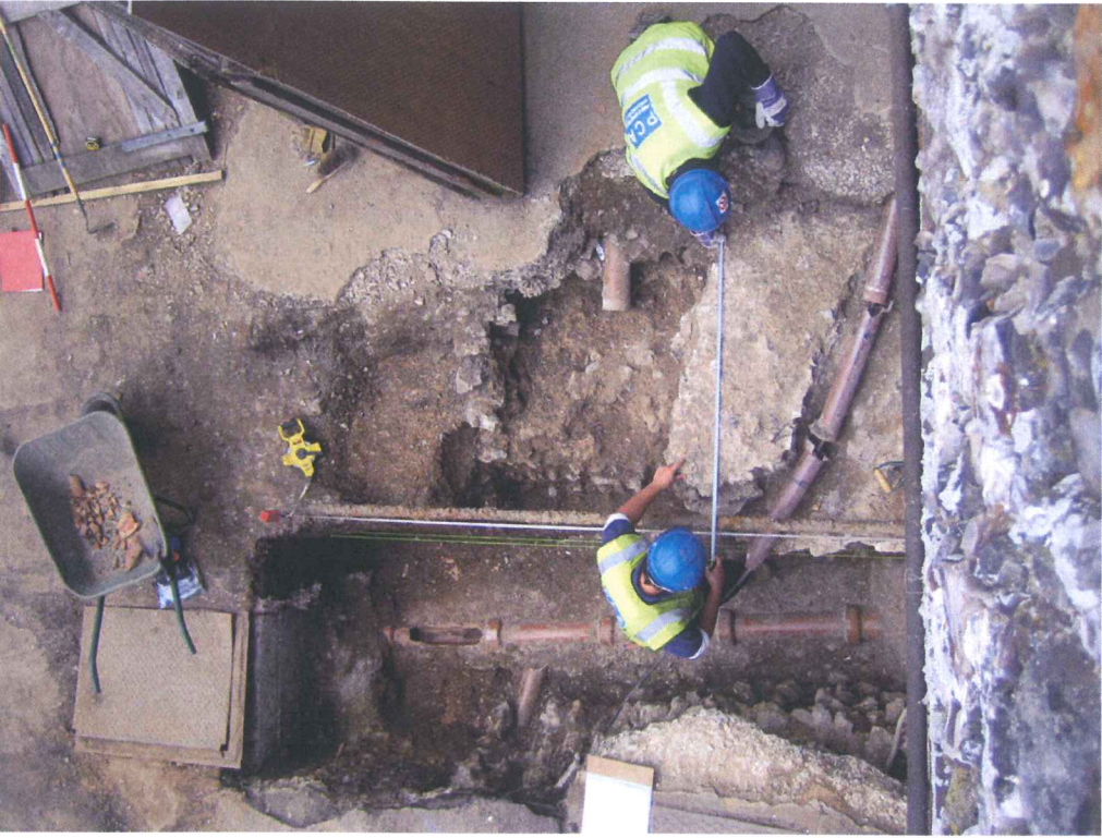
Plate 13: Civitas Wall (Area D; Phase 6; looking east from city wall)
